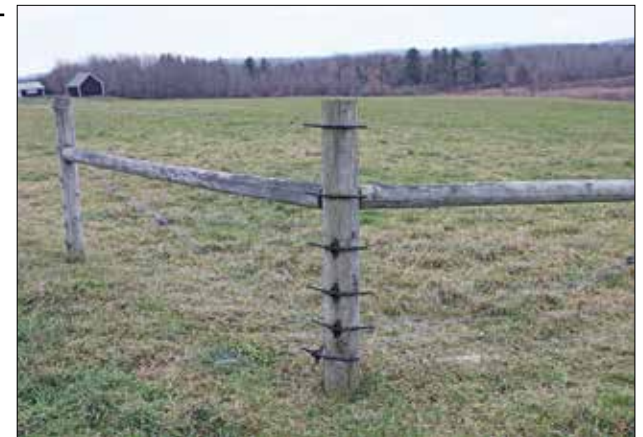
High tensile fences need strong corners and bracing. Rich Taber / CCE Chenango
