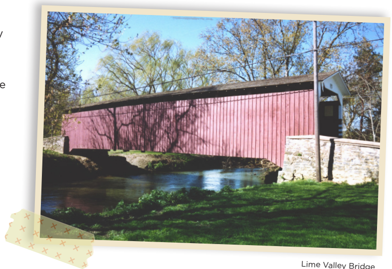
Lime Valley Bridge
