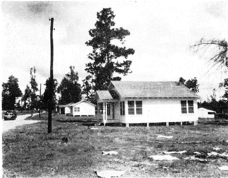
Shirley Daniel took the above picture across the highway from the Diboll Motor Company, looking north, to show some of the recently completed residence houses in the northeast part of town. These new houses, complete in every detail, are being built by Southern Pine Lumber Company for employees to improve the living conditions of our community and to make it the most modern and up-to-date town in this part of East Texas.
