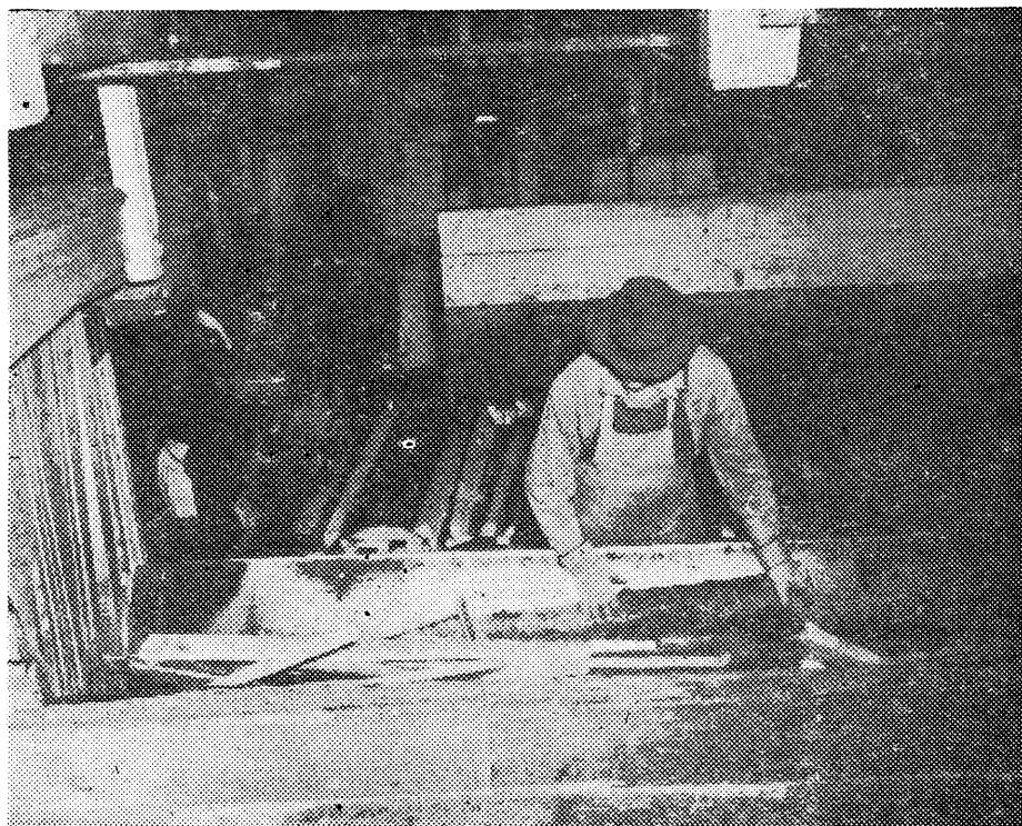
D. L. Helton selecting slabs and edgings in Southern Pine Lumber Company's Mill No. 1 at Diboll which will later be ripped into one inch squares 42 and 48 inches long for conversion into handles. These slabs and edgings, now made into a valuable product, were for many years considered waste.
