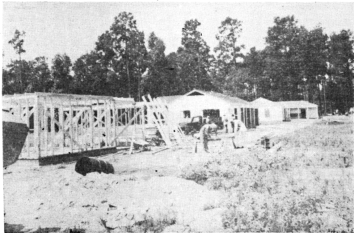
Above is a view of the six-unit housing project on the South side of Diboll which is being carried out by Southern Pine Lumber Company for its employees. The construction work is part of the Company's modernization program.
