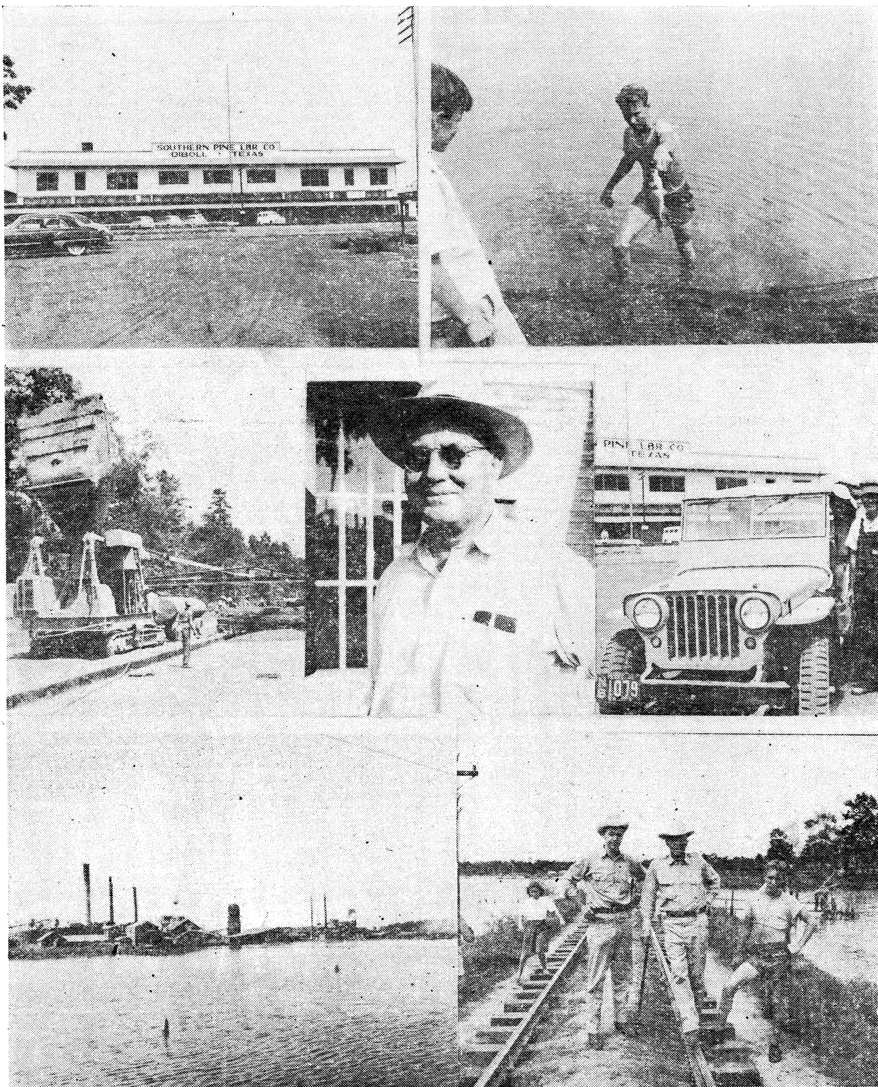
1. Shown at top (left) is Southern Pine Lumber Company's completely remodeled Diboll Store. 2. Left center: Paving machines at work on the concrete slab through town. 3. Bottom left: Look-
