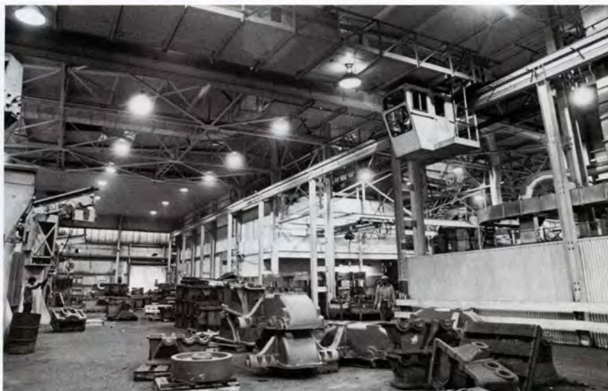
A new addition to the cleaning room is the overhead crane which moves large castings to and from the individual booths
