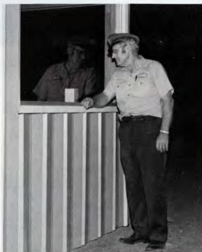
Ray McCollum, gate #11 second shift guard, checks the new guard house that is being built across from the welding shop
