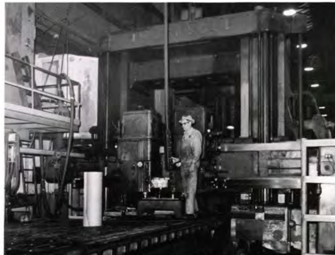
Avery Lee stands atop the adjustable rail Ingersoll milling machine which demanded full attention from the maintenance crew the last week of January for a semi-overhaul. It is the largest machine of its kind in the South, capable of machining an object 9 feet wide, 8 feet tall, 26 feet long. Because gear boxes go through this machine, it is vital to production
