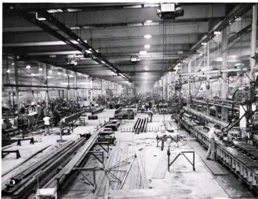
Most of this bay in the trailer plant is being used for structural work on components for the C-114D units. Other areas in the plant remain devoted to trailer building
