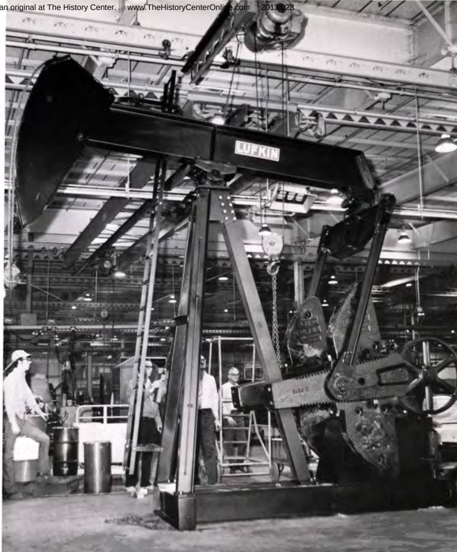
The first pumping unit completed by the Trailer Division employees is assembled and undergoes final testing. The unit was displayed outside the plant for several weeks
