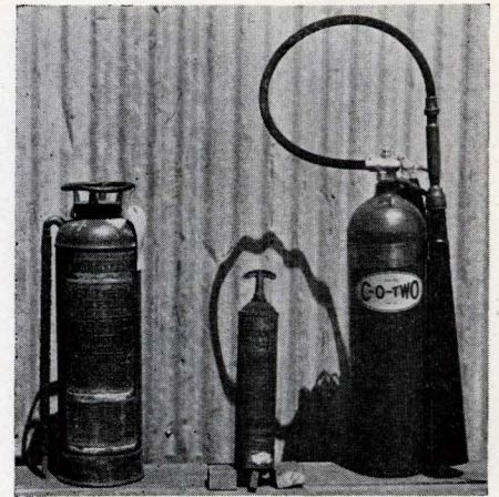
Here are pictured the three type extinguishers used here in the plant. Left to right: Soda-Acid, Pyrene (carbon tetrachloride) and carbon Dioxide (CO 2 ).
