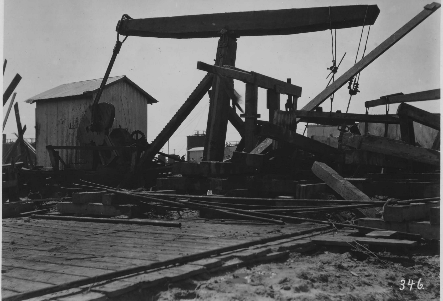
WIND STORM, PIERCE JUNCTION, APR. 21, 1927. GULF JACKSON #1. DERRICK BLOWN AWAY. NO DAMAGE TO UNIT, EXCEPT BENT PITMAN, WHICH HELD SAMSON POST AND BEAM FROM FALLING.
