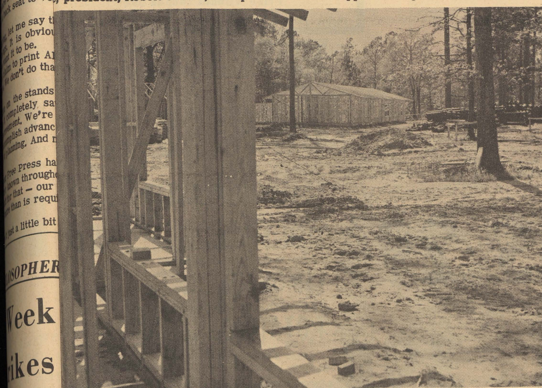
CO BUILDERS of Houston is moving along on construction of 80 new low-rent public housing units, just off South Street adjacent to the 120-unit Diboll.
