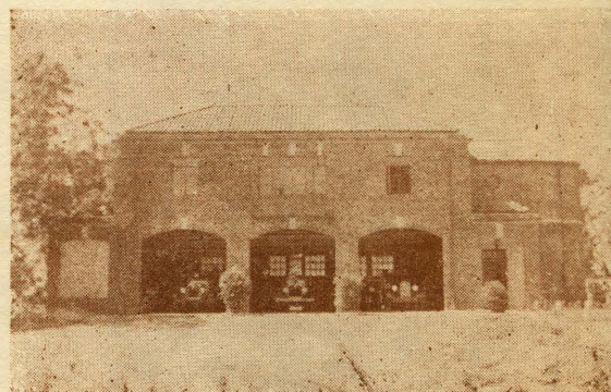
Lufkin Fire Station
