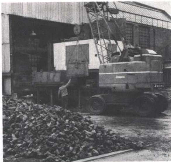
Fig.11 Use of mobile crane for material transfer.
