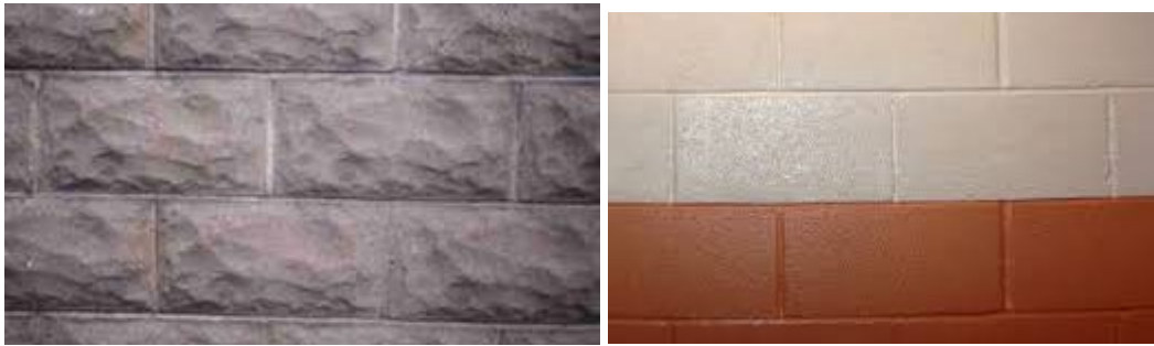
Figure 1 Finished concrete block is acceptable.
