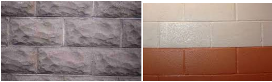
Figure 1 Finished concrete block is acceptable.
