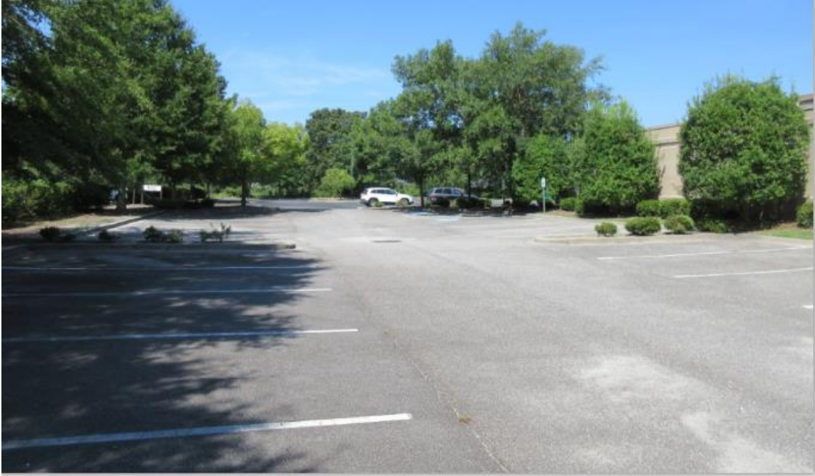
Parking Lot Facility
