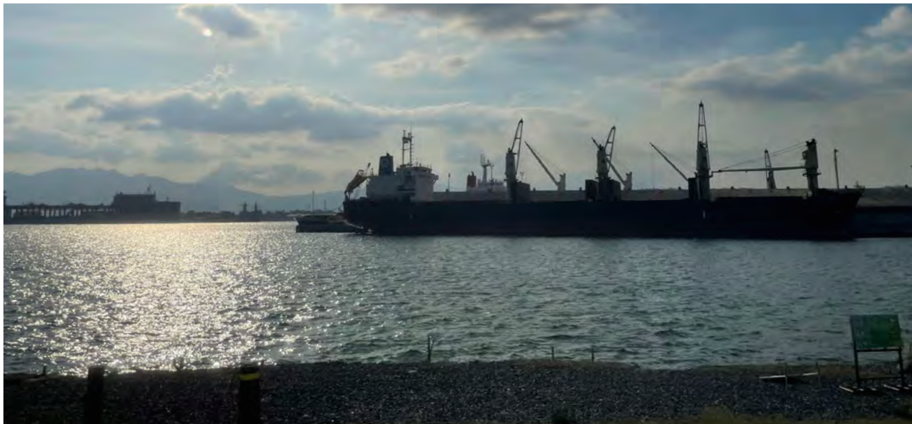
Pictured here is a shipping terminal five miles east across Subic Bay from the Hanjin Shipyard. When Hanjin went bankrupt in 2016, there was concern that the port would be acquired by a Chinese company with close ties to Beijing, but with the assistance of the U.S. Development Finance Corporation and Philippine President Rodrigo Duterte's administration, an American private equity firm acquired the shipyard. (Joshua Fitt/CNAS)
