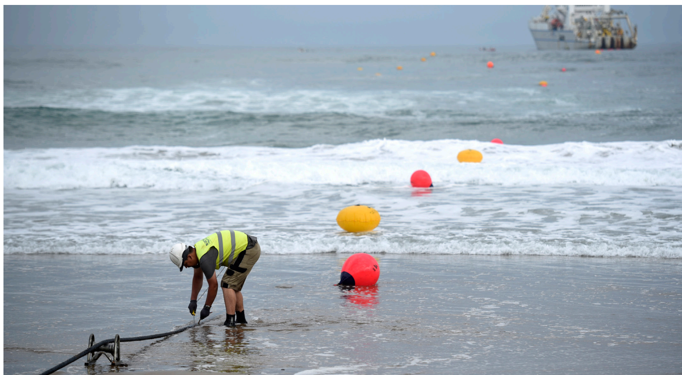
Technicians moor the Marea subsea cable near Sopelana, Spain. Financed by Microsoft and Meta, the 6,600-km link from Virginia to Bilbao illustrates how U.S. tech firms have become key drivers of subsea cable infrastructure to expand reliable, high-speed connectivity abroad. (Ander Gillenea/AFP via Getty Images)
