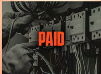
Lake Worth Electrical / HVAC Cost $265,000
