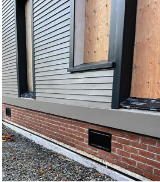
Penhallow-Cousins House c. 1750 on new wet-proof foundation with flood vents.
