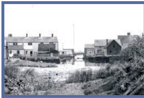
Puddle Dock before being filled in.
