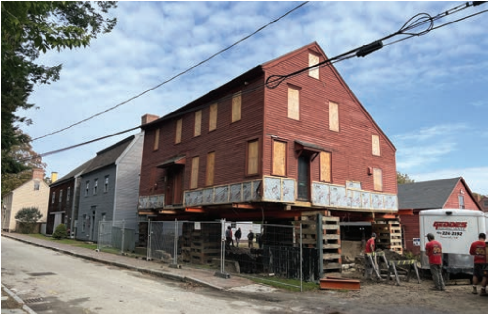
Penhallow-Cousins House on cribbing to replace its foundation.
