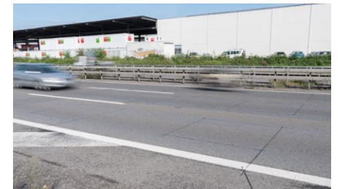
Induction loop within the road registers vehicle type and speed. Source: [6]
