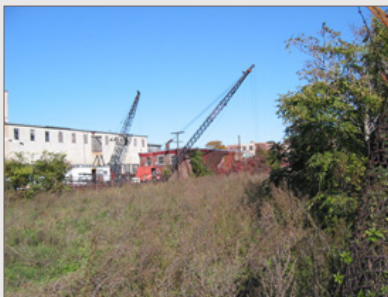
Carlton Wharf site - before
