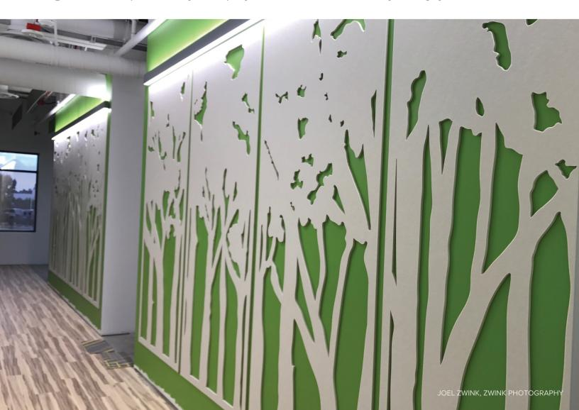
Kirei's EchoScreen was used to cover hard surfaces prone to reflecting sound. The screens effectively absorbed sound that would have otherwise been reflected off of the white walls, while other panels were suction-cupped onto glass walls, offering sound absorption as well as more privacy.
