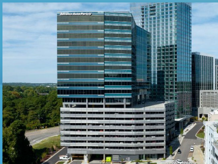
ADVANCE AUTO PARTS TOWER | RALEIGH
