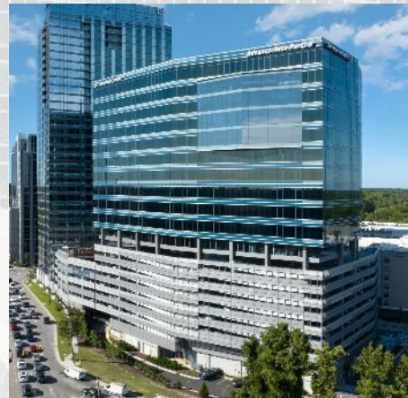
ADVANCE AUTO PARTS TOWER 2025 | RALEIGH
