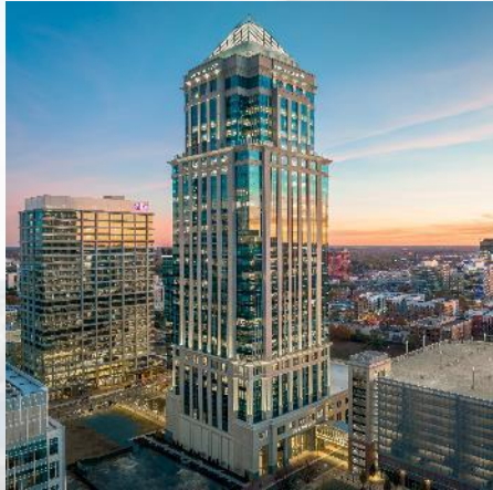
BANK OF AMERICA TOWER 2019 | CHARLOTTE
