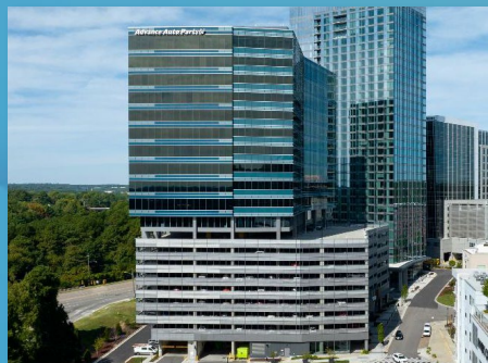
ADVANCE AUTO PARTS TOWER | RALEIGH
