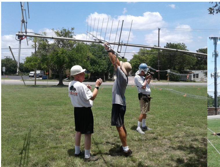
Here are the VHF/UHF antennas being erected on the N5MNW tower.
