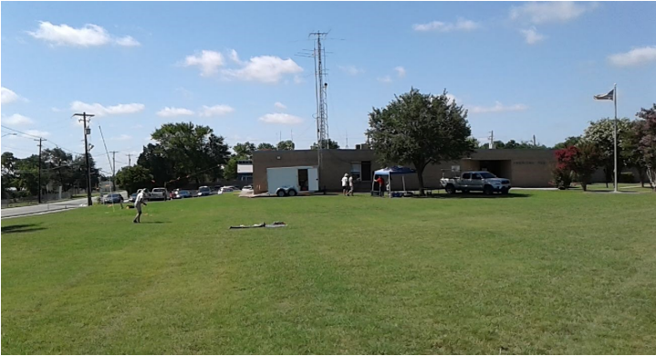
North side of the Red Cross location, facing south. Antennas are going up!
