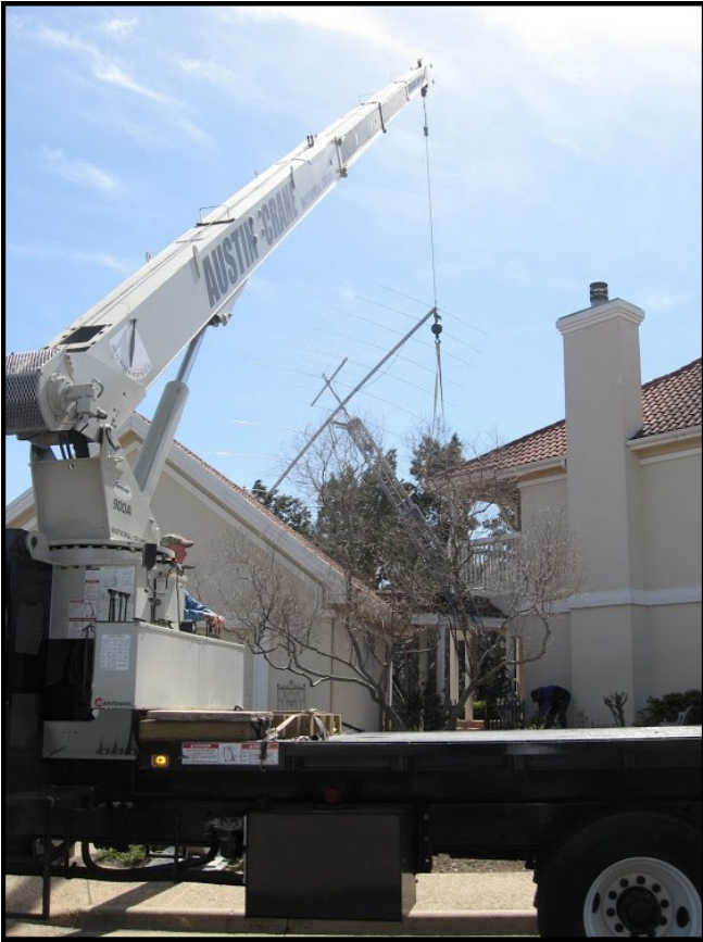
Here we see the crane lifting the entire tower with antenna still attached off the ground and a lot of thanks to the expertise of Larry and Terry.
