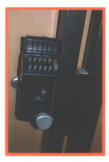
7. Completed Lock. Free Exit side . Keypad disengaged.
