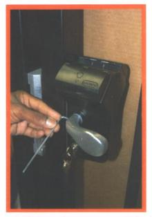
6. Tighten the set screw on the handle. We recommend using a "Loctite" type product on the screw to keep it from loosening in high traffic applications.
