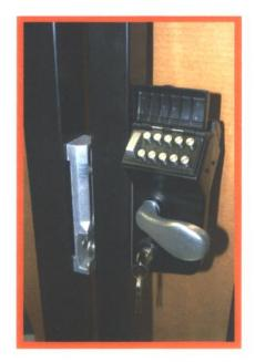
8. Completed Lock. Controlled Access side. Keypad and key access .
