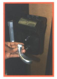
5. install the female half of the handle on the controlled access side of the gate.
