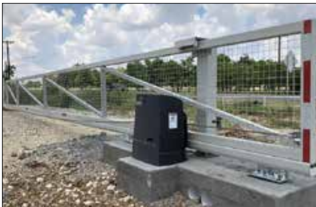
Aberdeen Gates, Weatherford, TX installed a security gate at a local Ford dealer. Model CGS-350.8P was used since the gate opening was large and the gate itself was quite heavy. The gate is fully automated.
