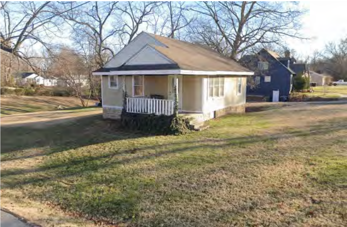
Age (85 Yrs.), Size (728 Sq.Ft.), Design (2BR-0BA), Stone Foundation, No Front Sidewalk or Driveway, No Public Sidewalks & Curbs & Gutters
