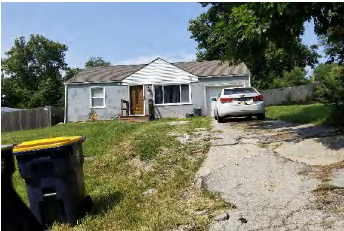
Unkept Landscaping (Golden Oaks)
