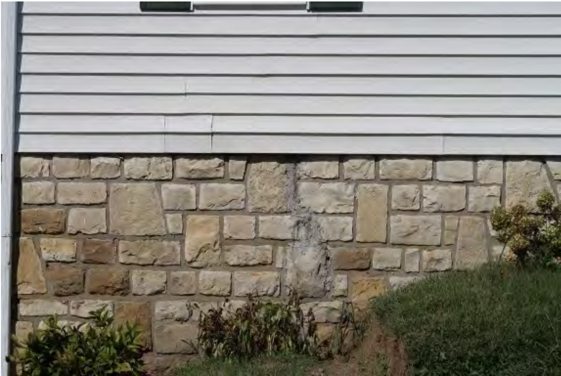
Stone & Mortar Foundation
