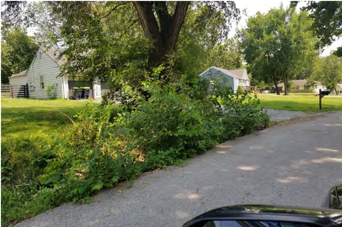
Excessive Weeds In Drainage Ditches (Antioch Acres)
