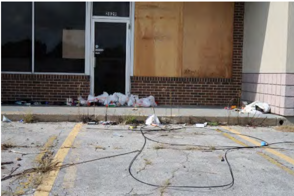
Illegal Dumping At Vacant Retail Building (2827, 2829, 2835 NE Vivion Road)
