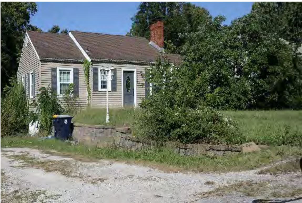
Unkept Landscaping (Golden Oaks)
