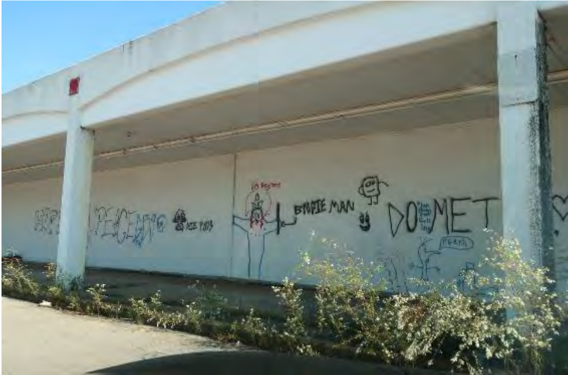
Graffiti And Weeds On The Kmart Exterior
