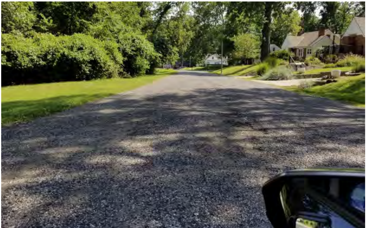
Gravel/Asphalt Chip Public Roadway – N Spruce Avenue (Fox Woods Subdivision)
