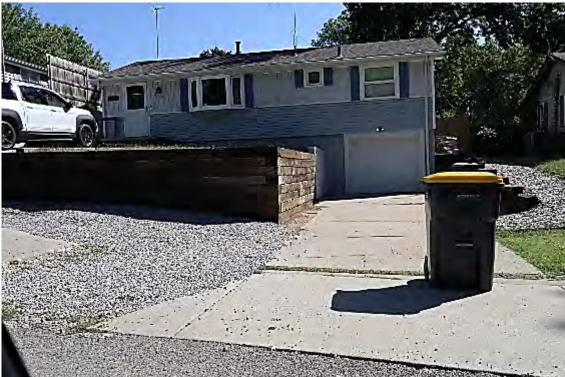
Unsecured Retaining Wall
