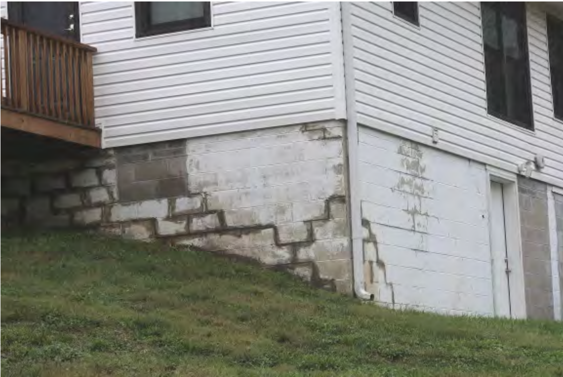
Concrete Block Foundation
