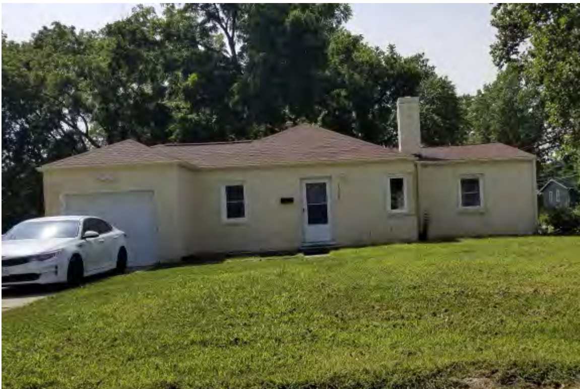
Unusual Design (Concrete Block Exterior), Minimal Windows, No Basement, Lack Of Public Sidewalks
