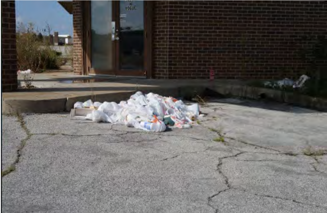
Illegal Dumping At Vacant Retail Building (2827, 2829, 2835 NE Vivion Road)
