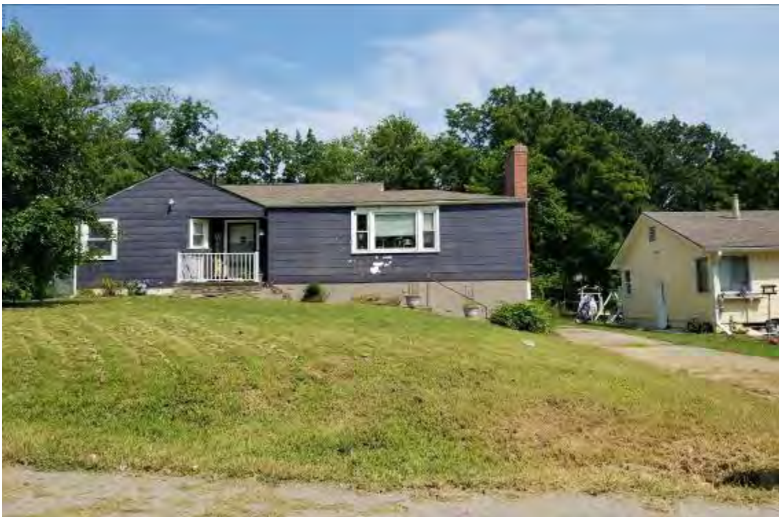
Potential Asbestos Shingle Siding, No Public Sidewalks & Curbs & Gutters
