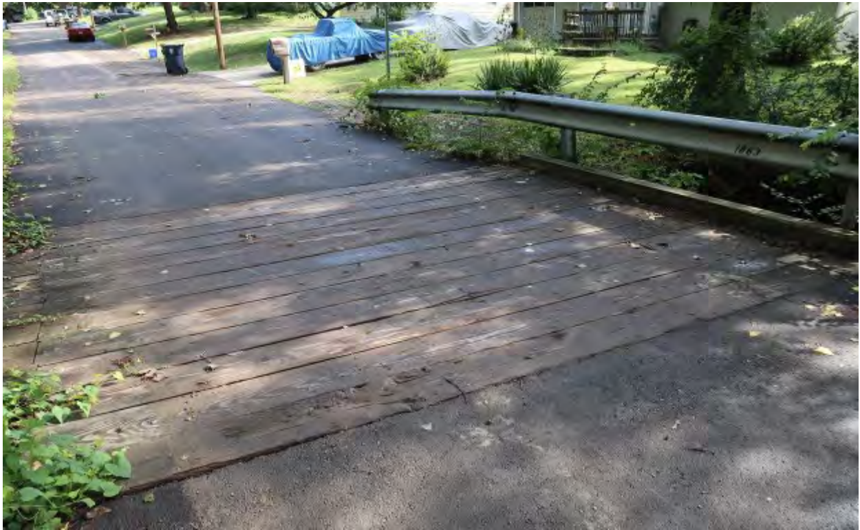
Wood Bridge On N Montgall Avenue In Golden Oaks
