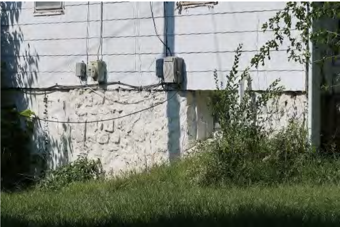
Stone & Mortar And Concrete Block Foundations
