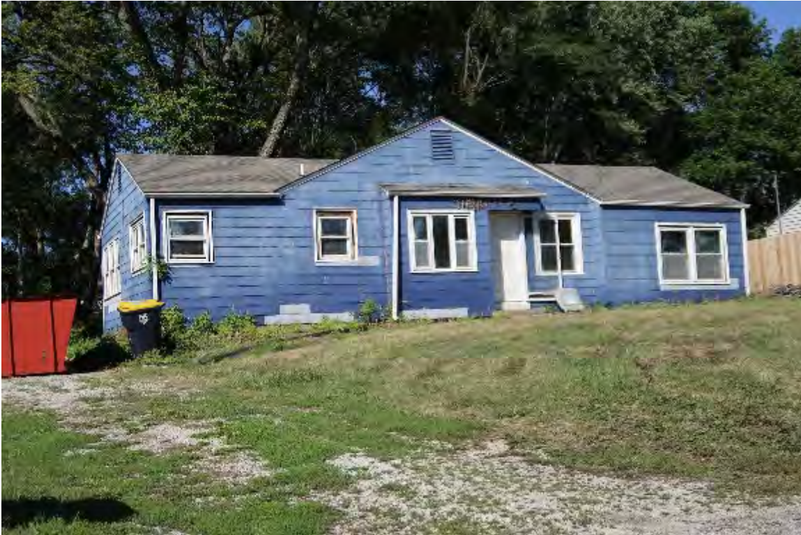
Unkept Landscaping (Golden Oaks)
