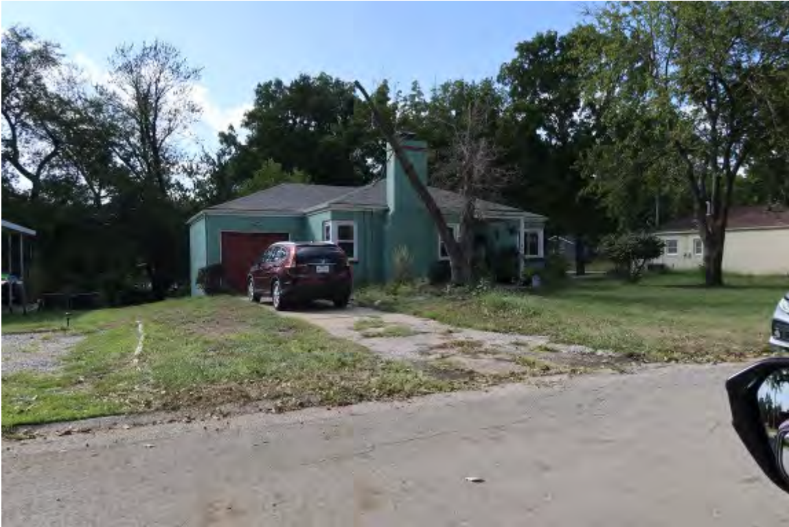
Unusual Design (Concrete Block Exterior), Design (2BR-1BA), Lack Of Public Sidewalks/Curbs/Gutters
