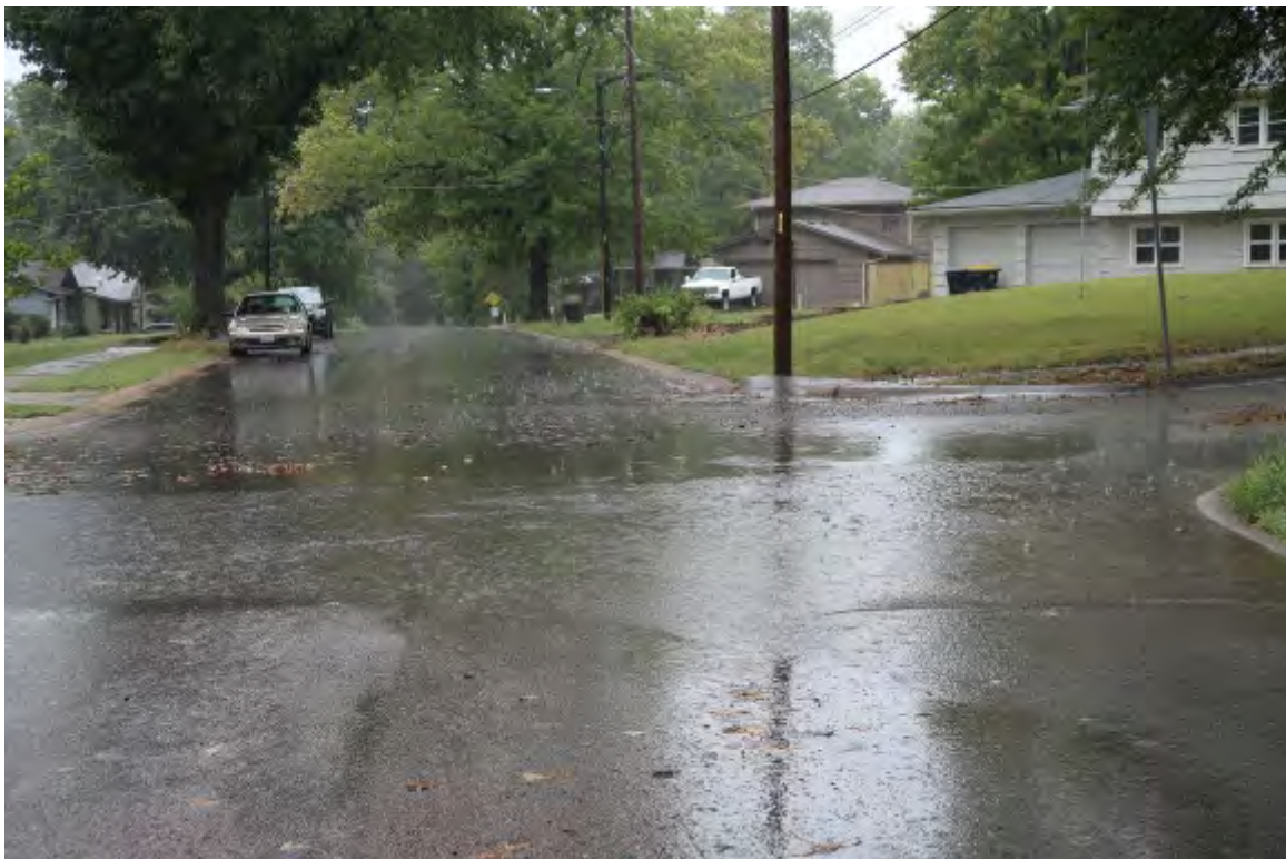
Poor Drainage In Glenhaven Subdivision
