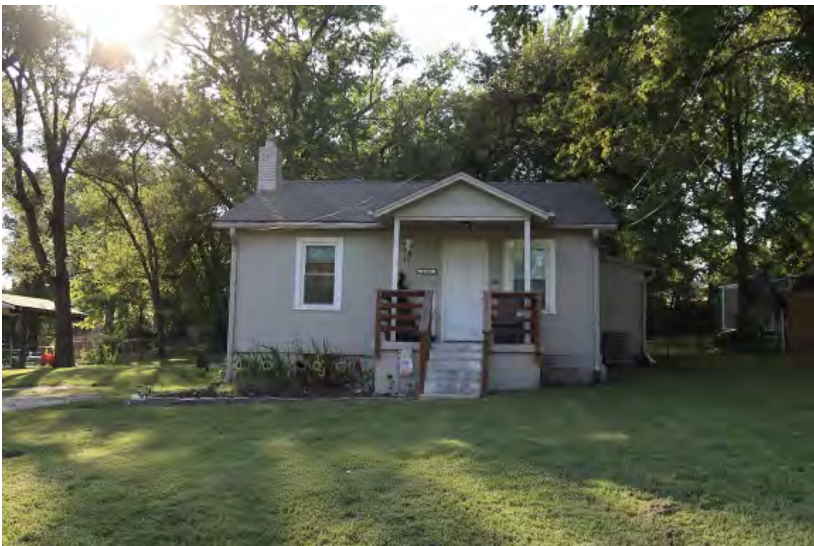
Lack Of Window Space
