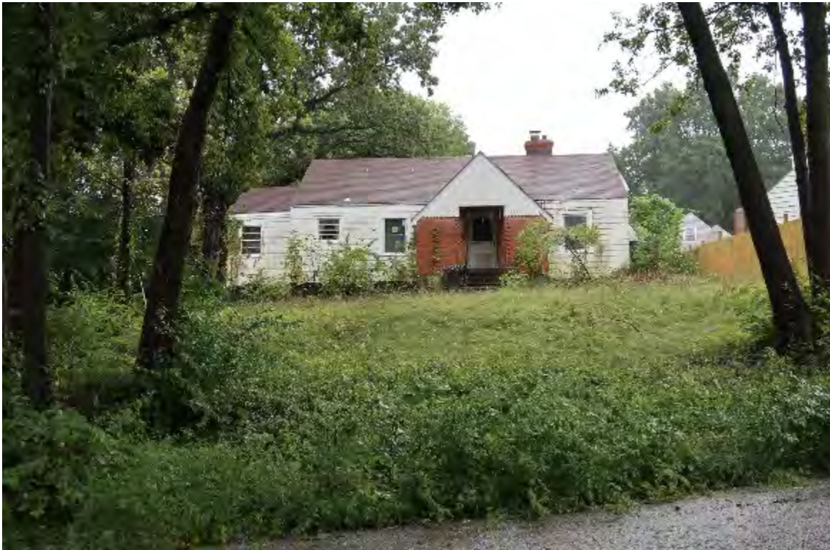
Excessive Weeds In Drainage Ditch (Fox Woods)
