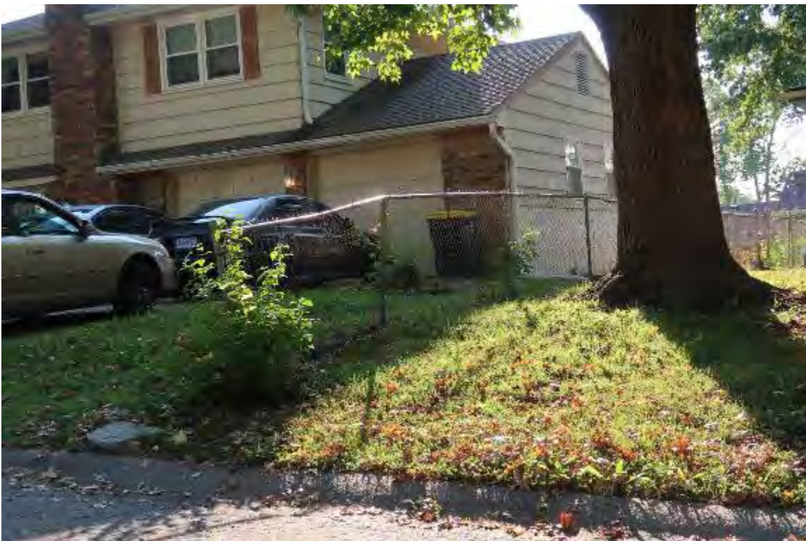
Deteriorating Fencing (Antioch Gardens)
