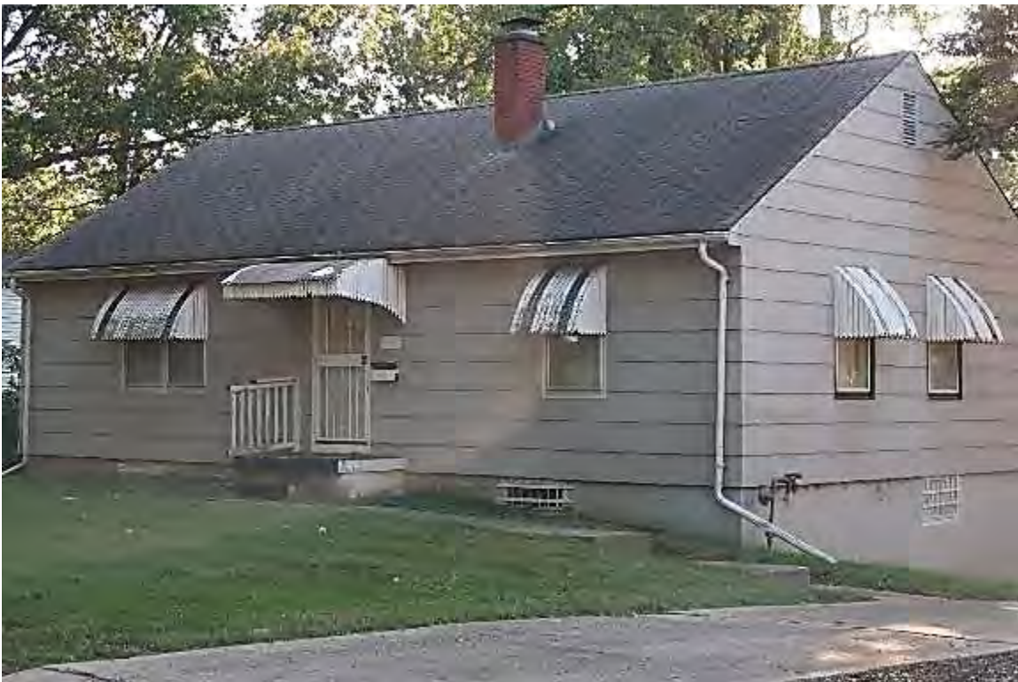
Potential Environmental Issue – Asbestos Shingle Siding
