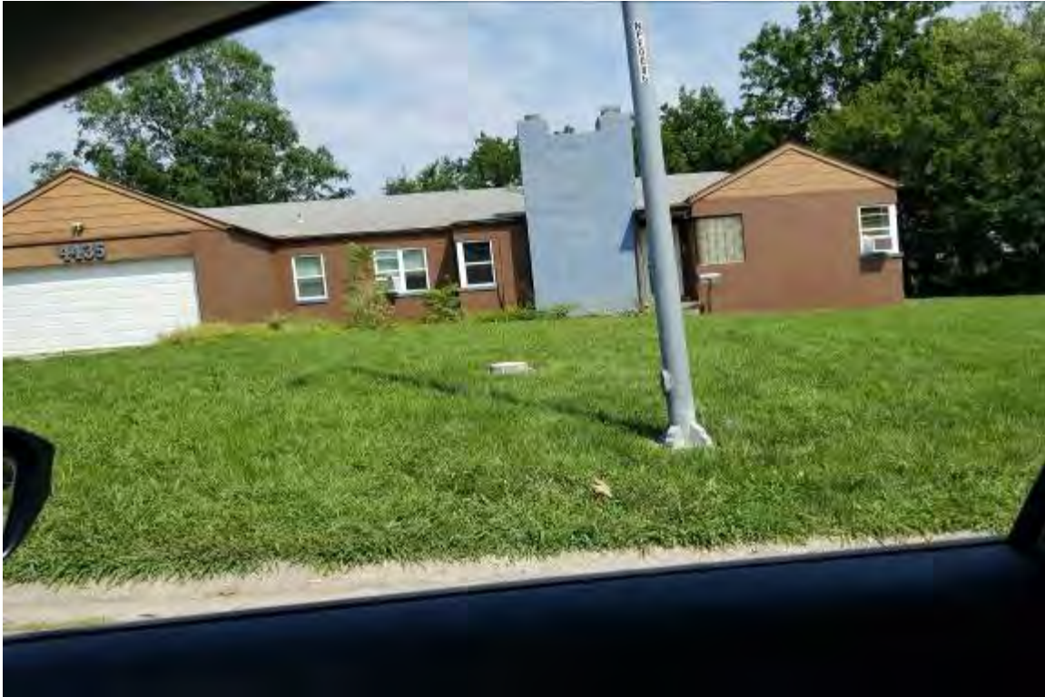
Unusual Design (Concrete Block & Glass Block Walls), No Central Cooling, Manhole/Streetlight In Front Yard
