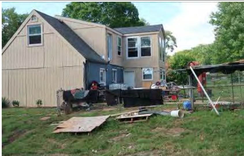
4425 Askew Avenue South (Road) Elevation
