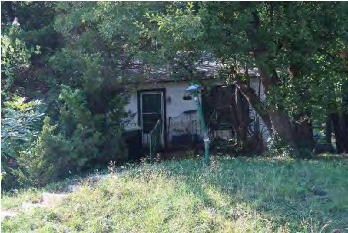
Unkept Landscaping (Golden Oaks)
