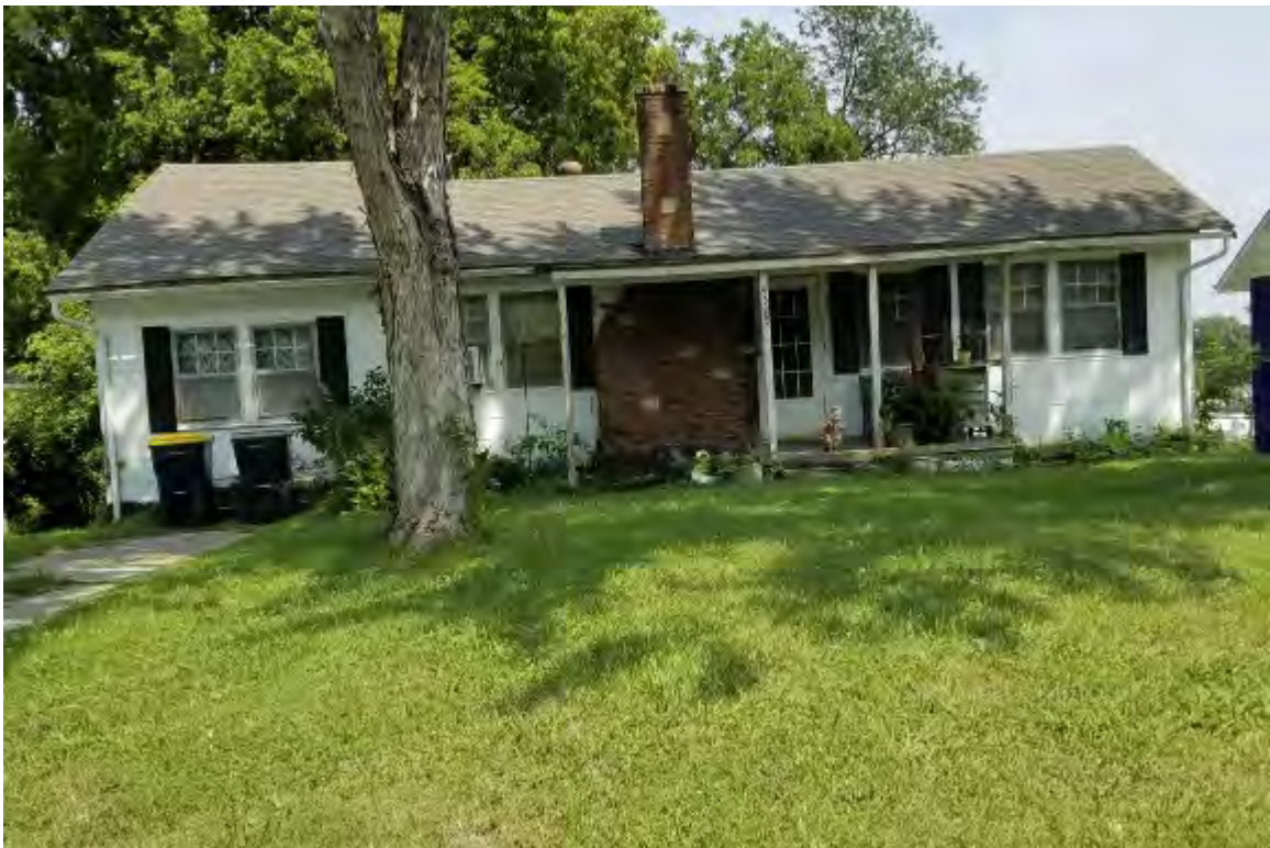
Lack Of Roof Gutters, No Garage, No Public Sidewalks/Curbs/Gutters
