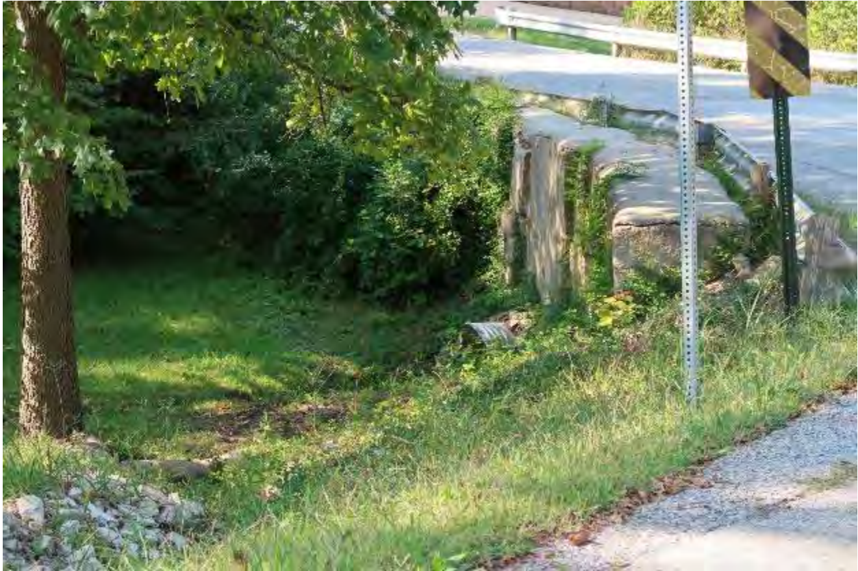
Open Drainage In Fox Woods
