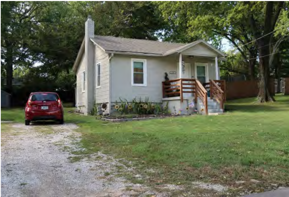
Age (125 Yrs.), Design (2BR-1BA), No Basement, No Garage, Gravel Driveway, Stone Foundation, Minimal Window Provision, No Public Sidewalks / Curbs / Gutters
