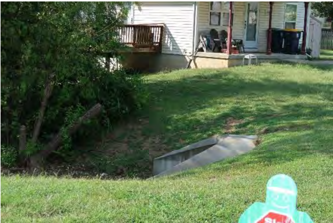
Open Drainage In Brookwood Heights
