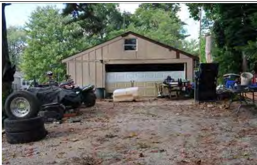
4425 Askew Avenue Free Standing Garage
