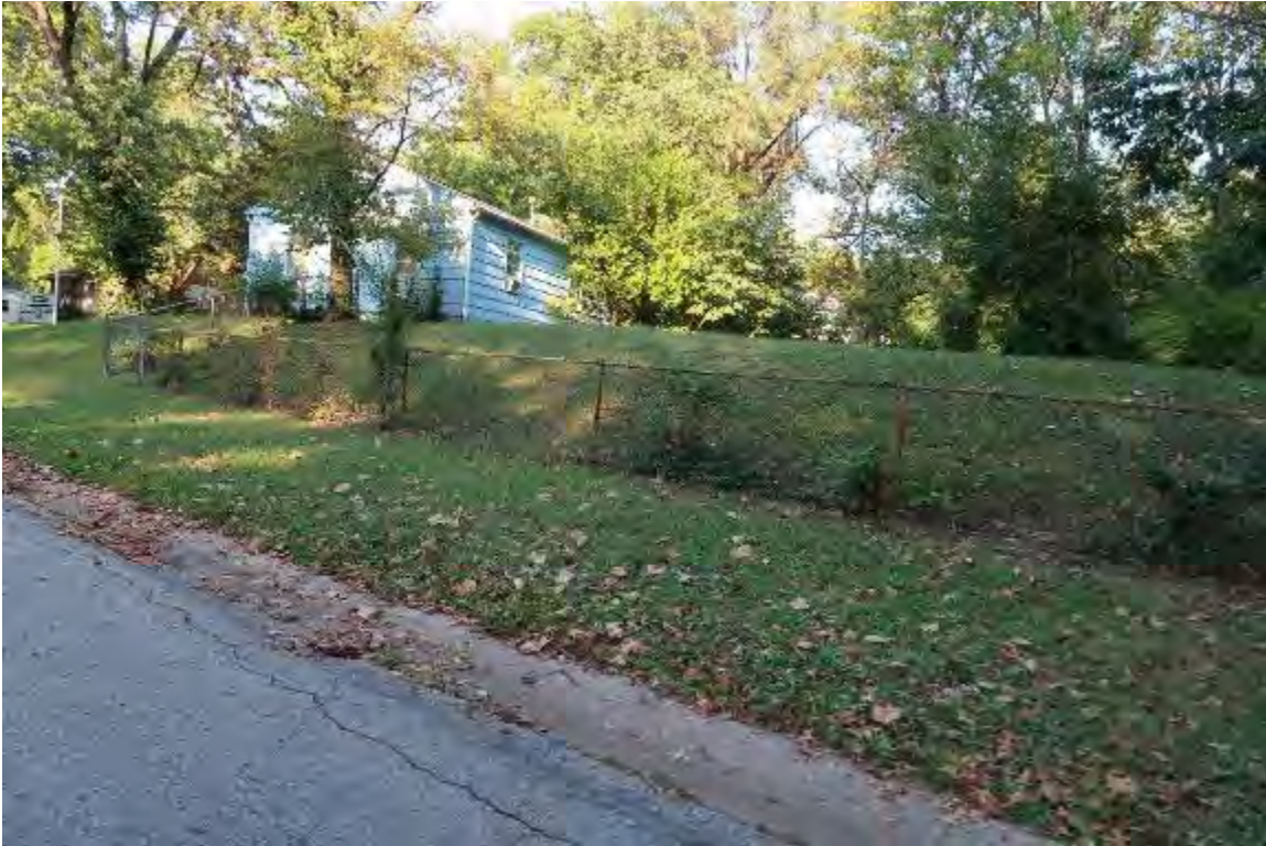
Deteriorating Fencing (Edgewood Acres)
