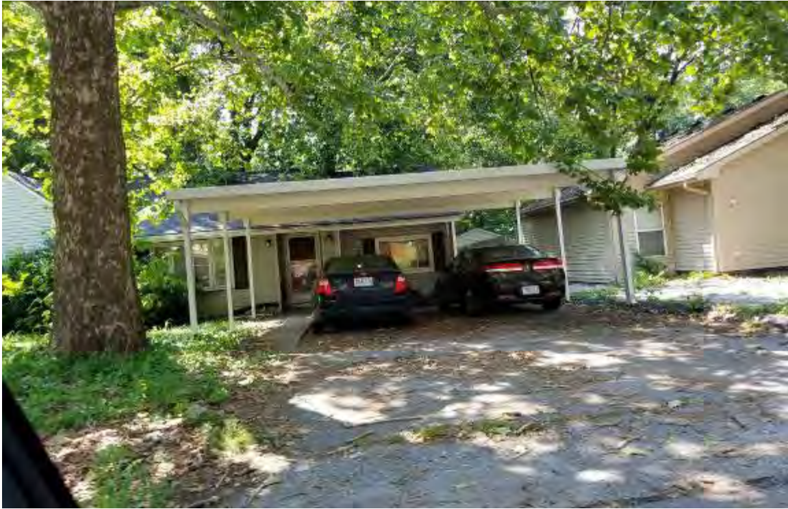
Obsolete Design (3BR-1BA), No Garage, Missized Carport, No Public Sidewalks & Curbs & Gutters
