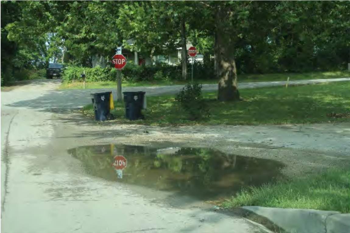
Standing Water Adjoining Sewer Inlet Due To Lack Of Curbs & Gutters To Channel Water Flow
