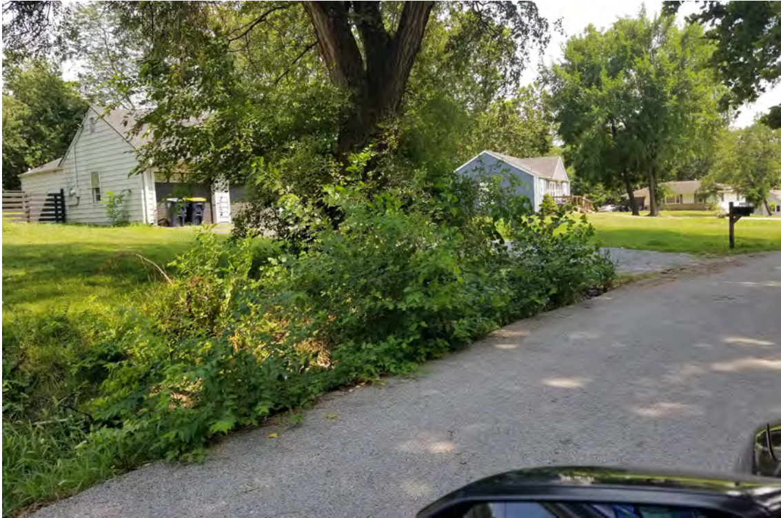
Excessive Weeds In Drainage Ditches (Antioch Acres)
