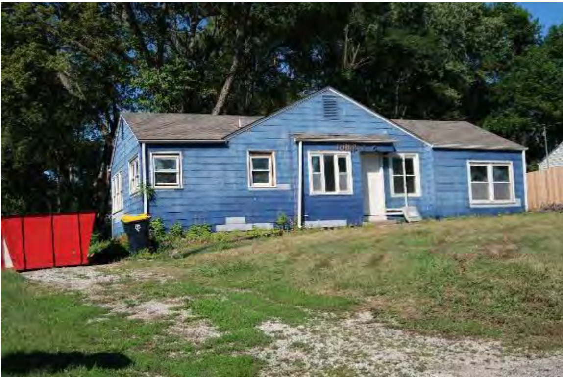
Deterioration (Golden Oaks)
