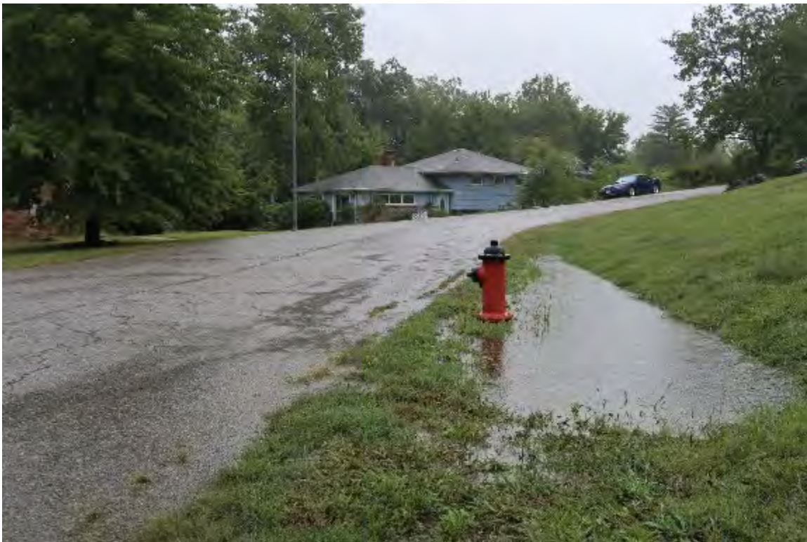
Standing Water In Drainage Ditches (Fox Woods)
