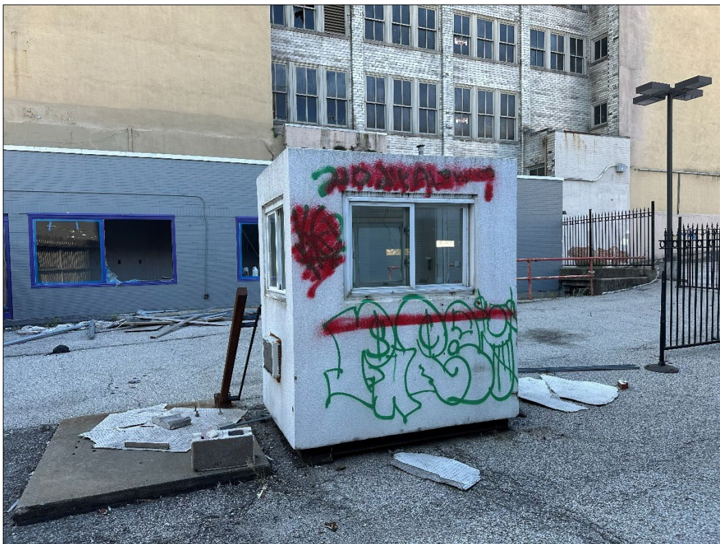
800 Grand Blvd – looking south – graffiti; broken window; trash/debris
