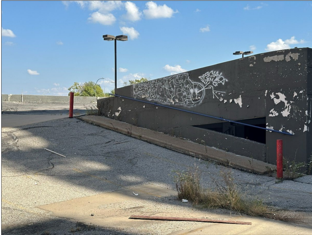
800 Grand Blvd – looking northeast – graffiti; overgrown vegetation; trash/debris
