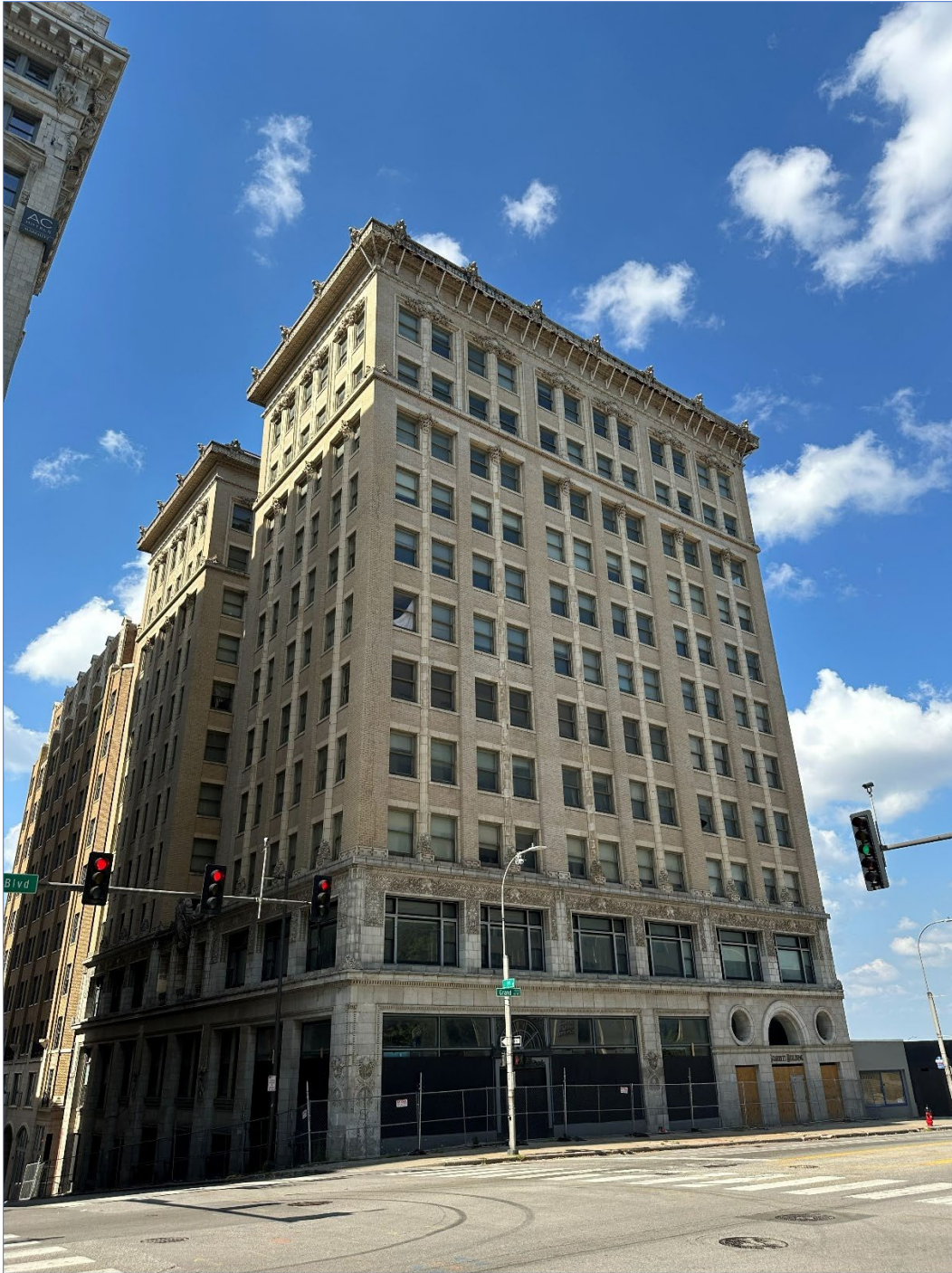
818 Grand Blvd (Scarritt Building) – looking northwest
