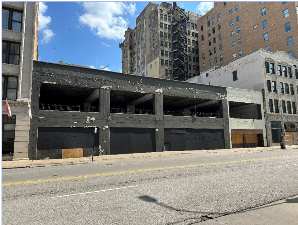
800 Grand Blvd (Walnut Entrance) – looking east; Scarritt Arcade on south side (right)
