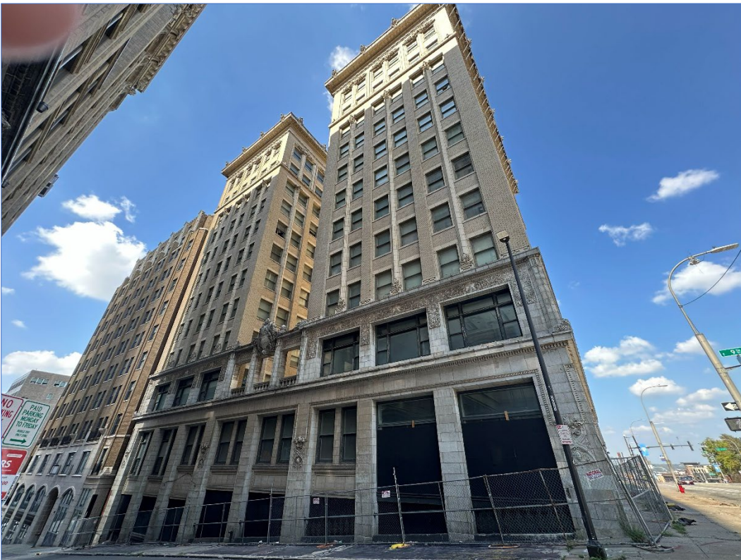
818 Grand Blvd (Scarritt Building) – looking northwest
