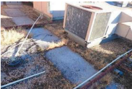
Organic growth Building 18/Block L
