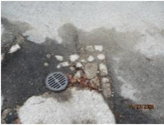
Parcel 12-14/Block C Garage Roof
