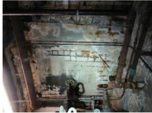
Basement Building 19/Block L
