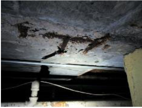
Subgrade Building 3/Block N
