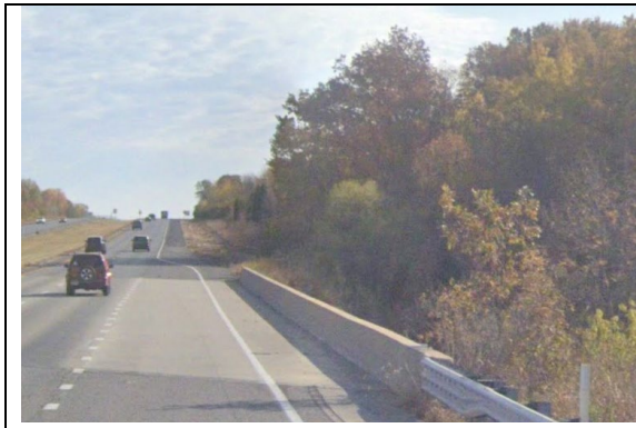
MO 152 facing east
