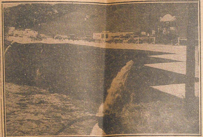
HUNGRY FLOODTIDE —Voracious flood waters recede after "biting" away huge piece of land, breaking up concrete of Ventura blvd. outside Los Angeles. (AP Wirephoto)
