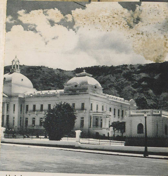
able in beauty and modernity with our own public buildings National Palace at Port-au-Prince, Haiti's capital city.
