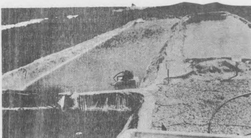
WRAP SYSTEM uses facultative pond (upper right) where algae assimilate degraded organic material in wastewater. It then flows into aerobic pond (center) and finally to decarbonation pond (lower left).
