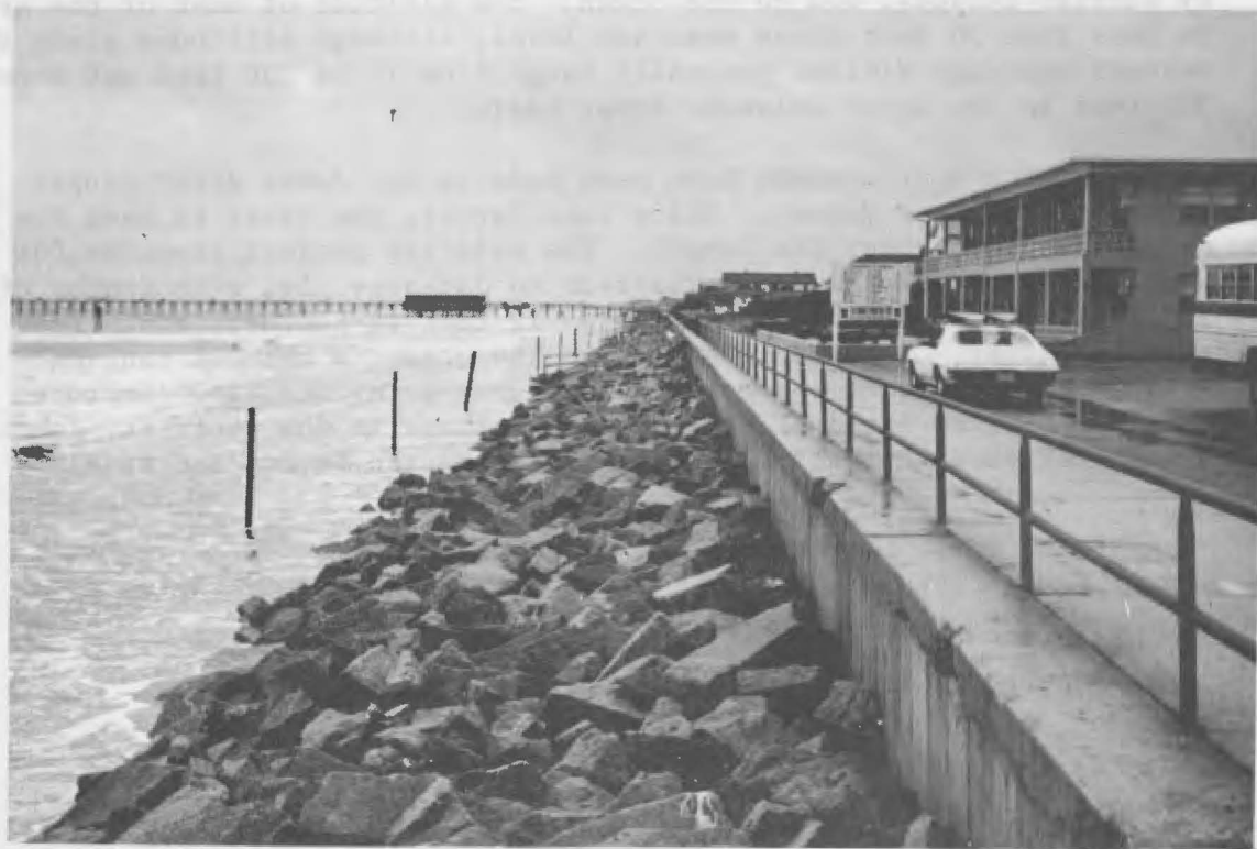
Jacksonville Beach (Duval County) - Problem beach, showing temporary stone revetment provided with Office of Emergency Preparedness funds (1971)
