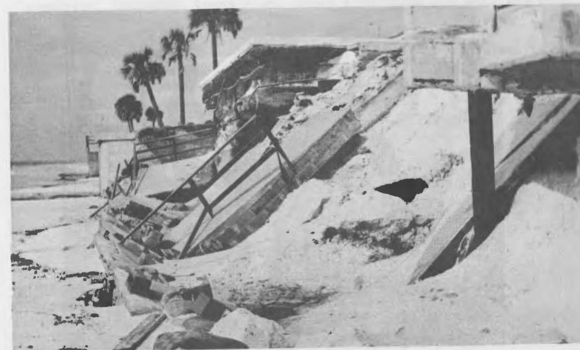
Panama City Beach Erosion - Damages to motel at Panama City caused by collapse of a bulkhead in the fall of 1970 following a week of sustained southeasterly winds
