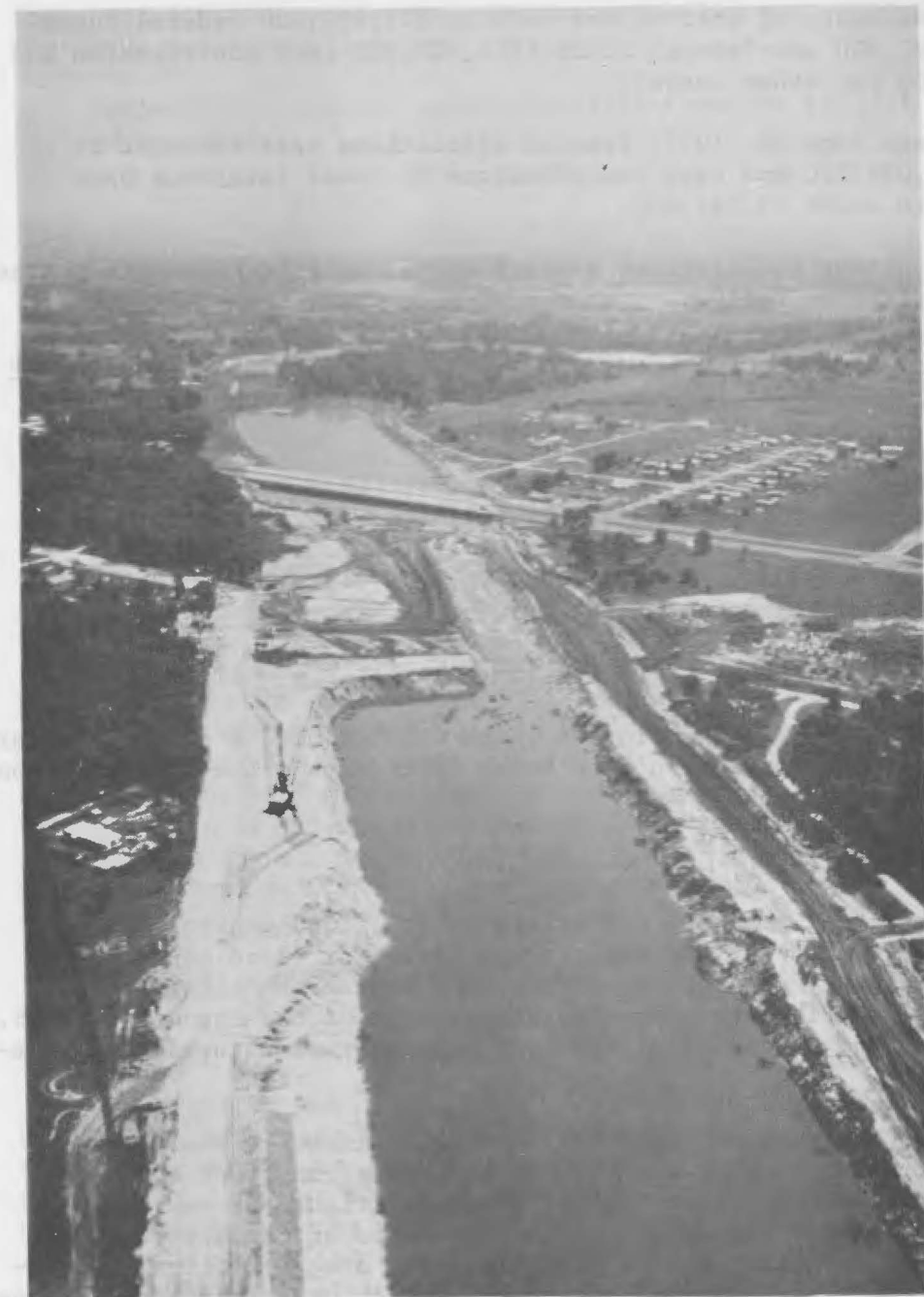
Tampa Bypass Canal under construction. Floodwaters from Hillsborough River eventually will move to the Gulf of Mexico via the Tampa Bypass Canal. View is northeast with new Highway 301 bridge in center of photo (August 1972)
