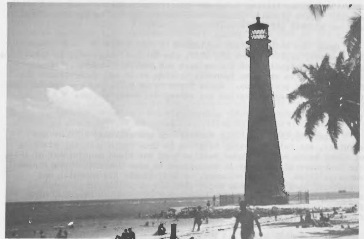
Cape Florida Lighthouse at Key Biscayne. This is one of the oldest structures in South Florida and was in danger of being undermined (1970)
