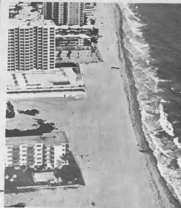
← Pompano Beach (Broward County), Fla. North end of project before construction (1970)
