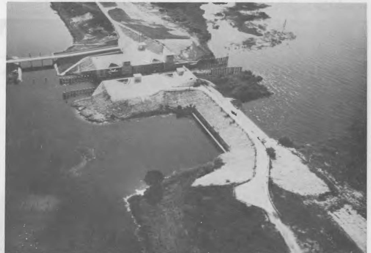
Conversion of Hurricane Gate Structure 6 into Lock Structure 193. View shows southern entrance of Taylor Creek (left) into Lake Okeechobee (right)
