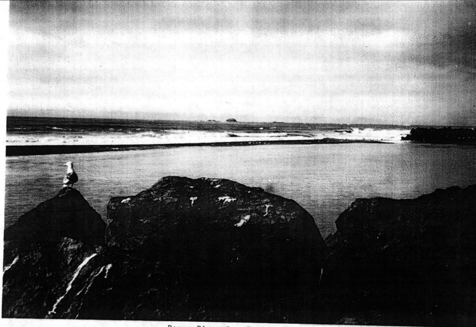
Rogue River Bar Sanded in Between North and South Jetties 1997
