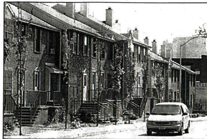
New development: Public housing is being built in the form of town houses instead of high rises near downtown Newark.
