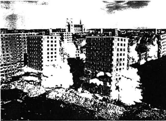
Demolition in Newark.
