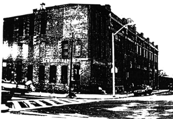
Demolition in Baltimore's Sandtown-Winchester.
