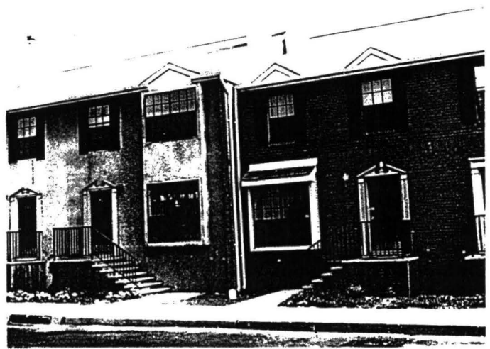
New townhouses on site.
