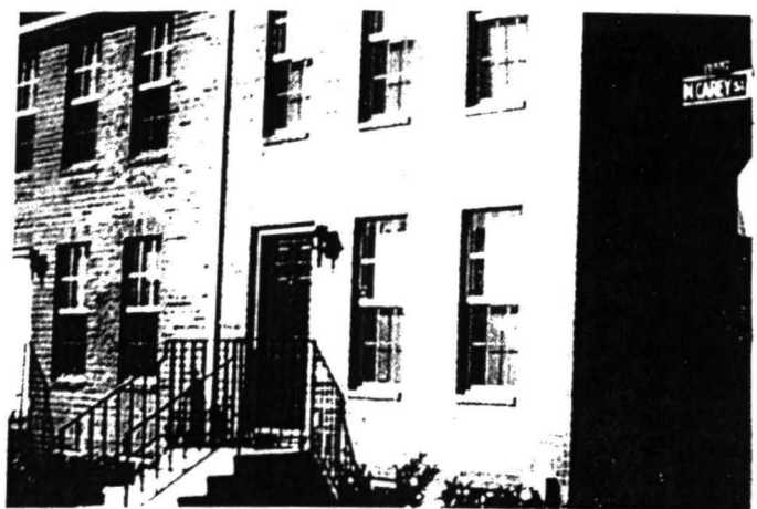
New townhouses on Baltimore site.
