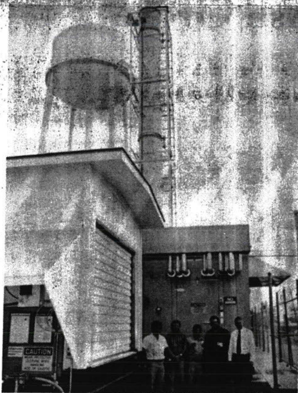
The scrubber at Baxter Healthcare Corp. in Mountain Home uses a high-efficiency process that reduces ethylene oxide emissions by 95 percent.
