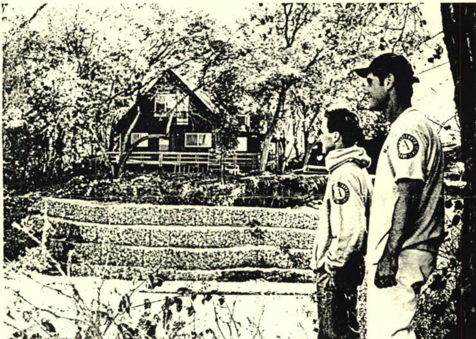
James Newman and James May (l to r) helped build the gabion baskets to protect this house on Auburn Ravine.
