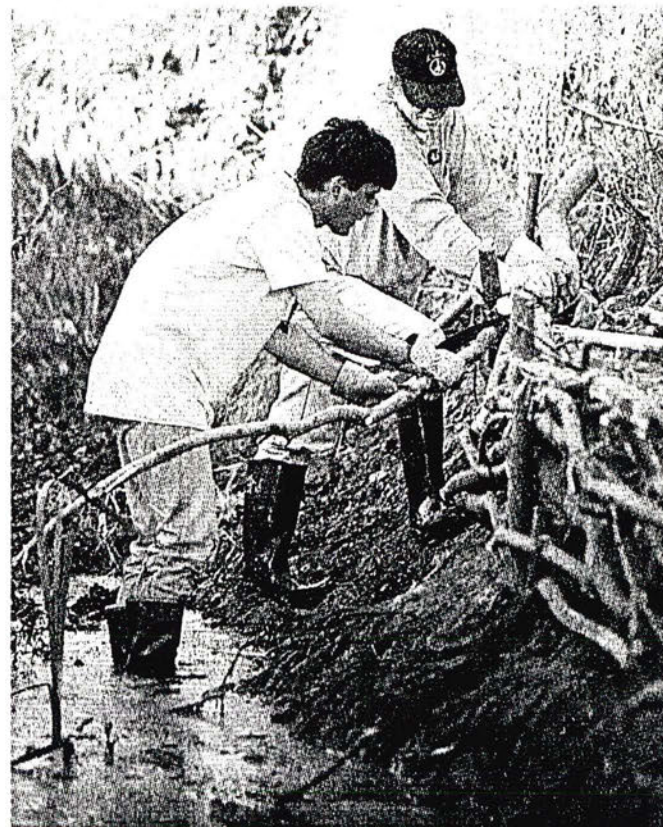
Americorps worker Chris Auld of Lakeport, left, and Stephanie Carey of Petaluma weave tree branches into a retaining wall built along an eroded section of Stemple Creek.
