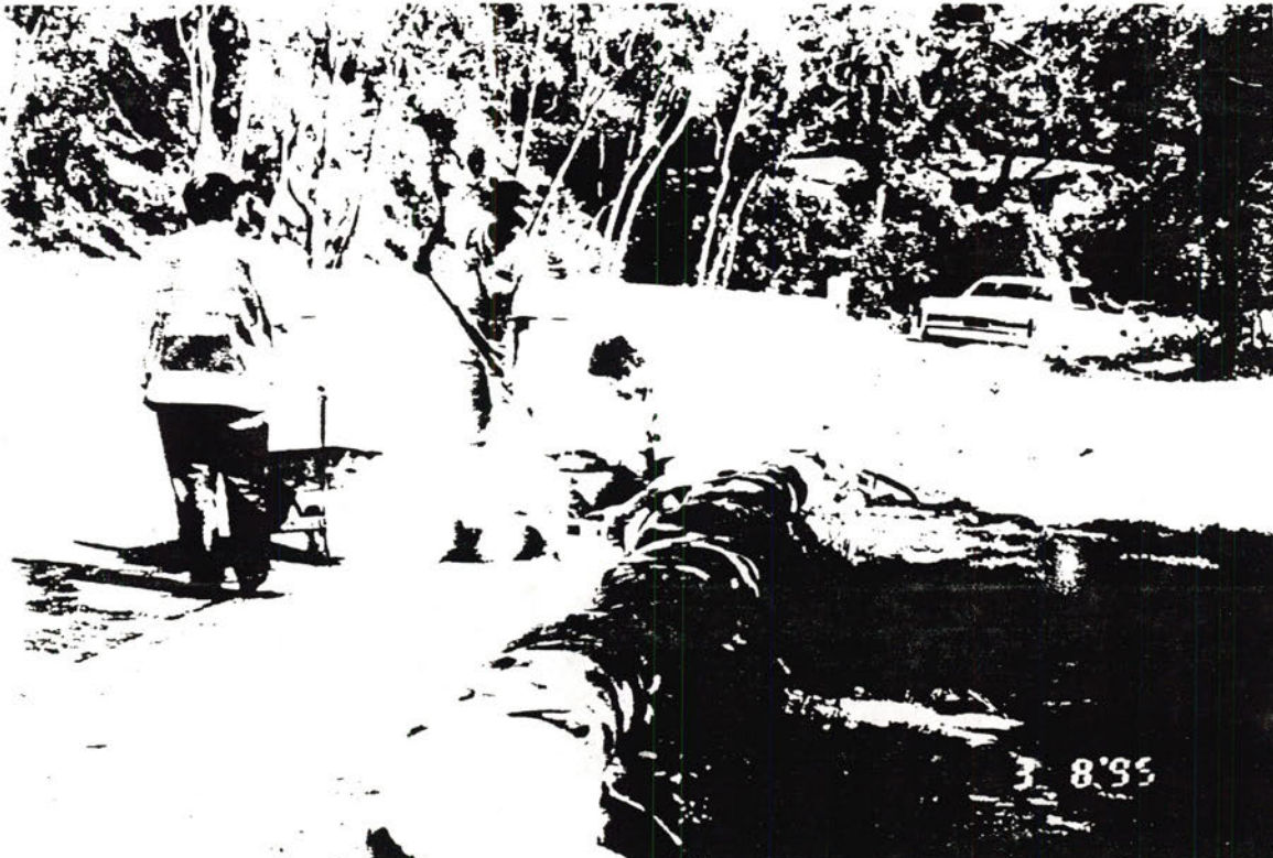
April Jurgen, Sandy Haynes, and Phillip Sam building a row of sandbags to protect a Pasadena resident from the mud and debris that flow down Loma Alta Drive. 3/8/95
