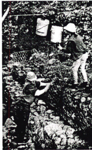
Members Installing Gabions to Stabilize a Stream Bank
