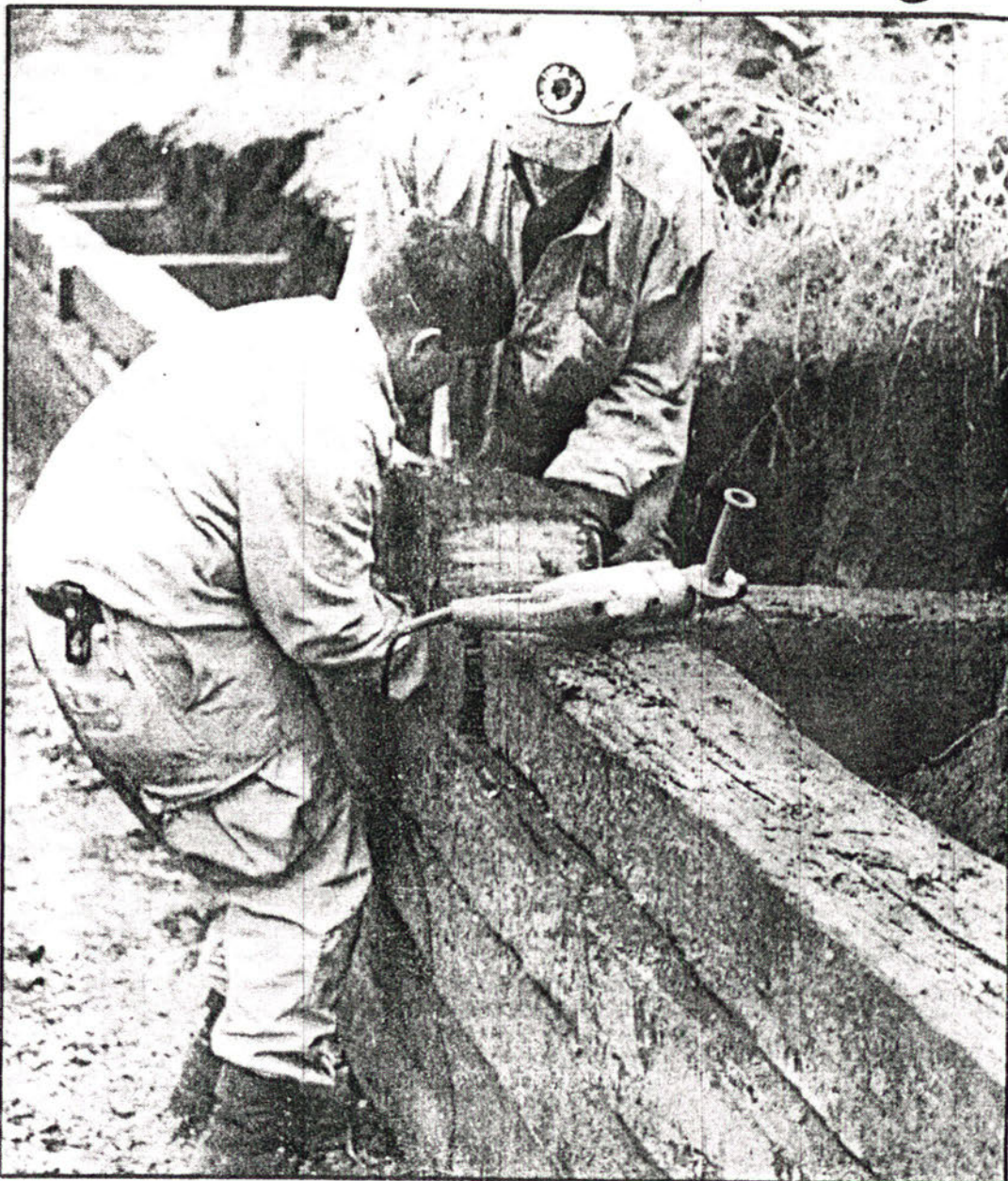
AMERICORPS IN ACTION — Brent Force (left) and Carl Lampman were two team members from the AmeriCorps Program who were working recently on a new retaining wall at Columbia Gorge Community College. Both work through the Northwest Service Academy's Mt. Adams Center. (Staff photo by Tom Stevenson)
