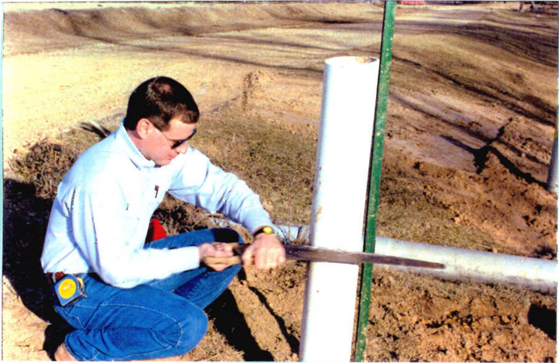
John Tom Murray, USDA/AmeriCorps Member - Dry Fire Hydrant Project, Winnsboro, Louisiana, cutting pipe to proper height.
