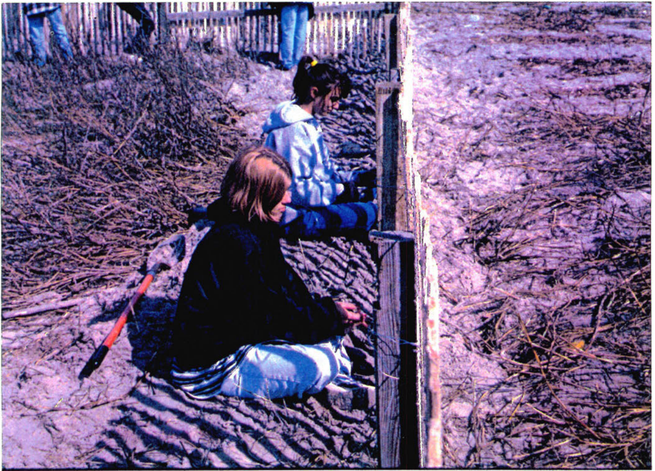
Louisiana Coastal Wetlands Environmental Corps Team Members constructing sand fencing.
