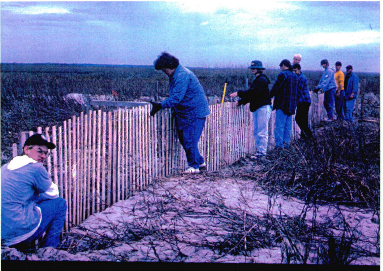
Louisiana Coastal Wetlands Environmental Corps Team Members constructing sand fencing.
