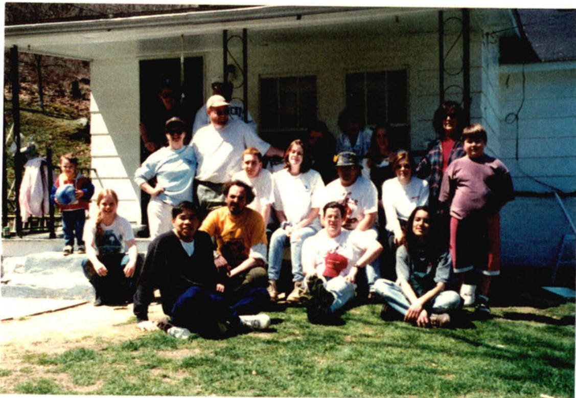
R21H: Volunteers stand in front of house they helped repair
