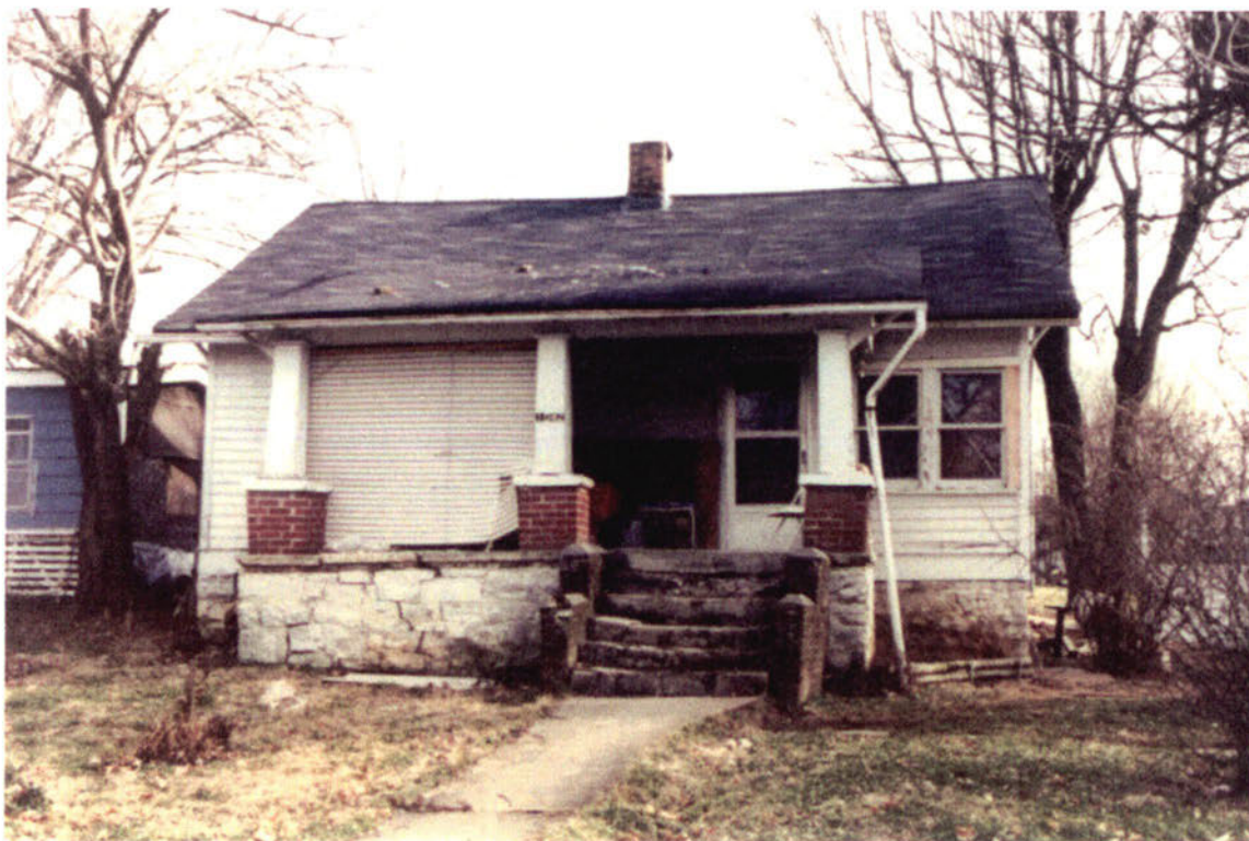
R21H: House before and after
