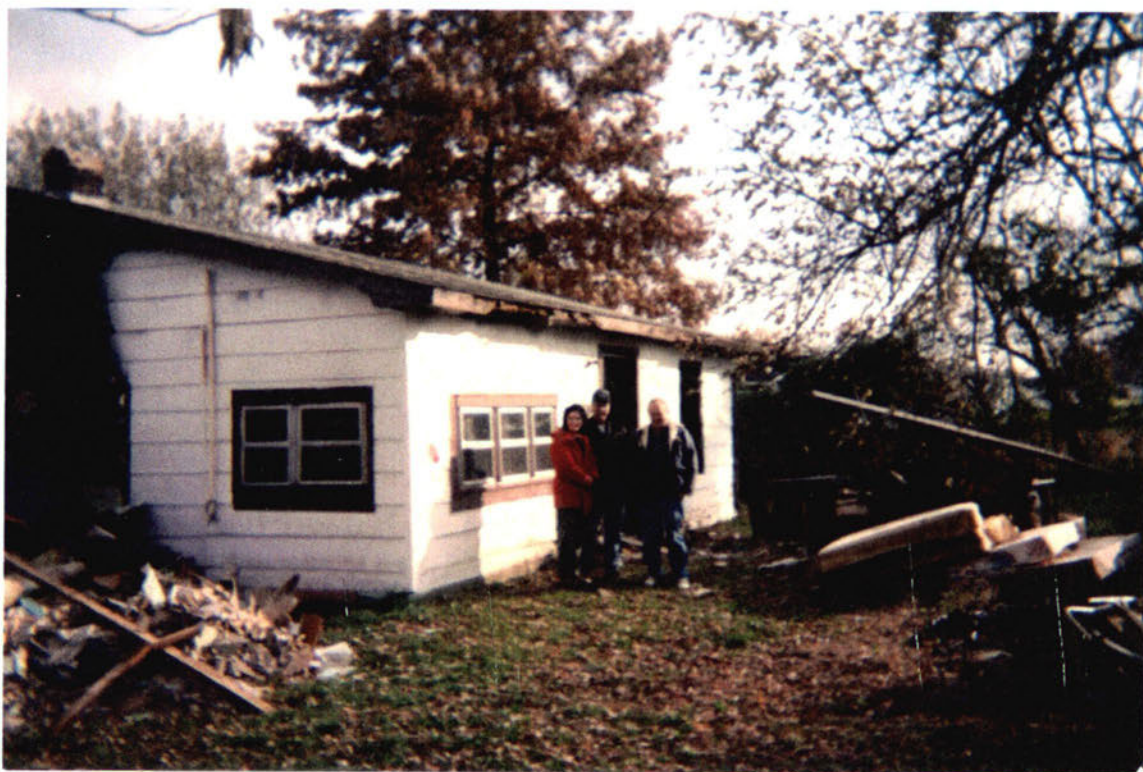
Burned house before
